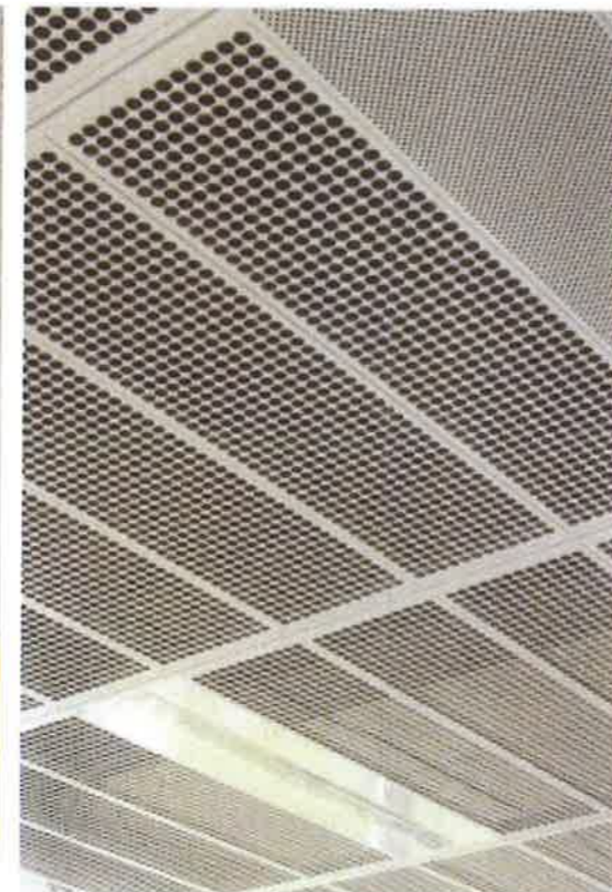
Metal pan ceiling to homebases
