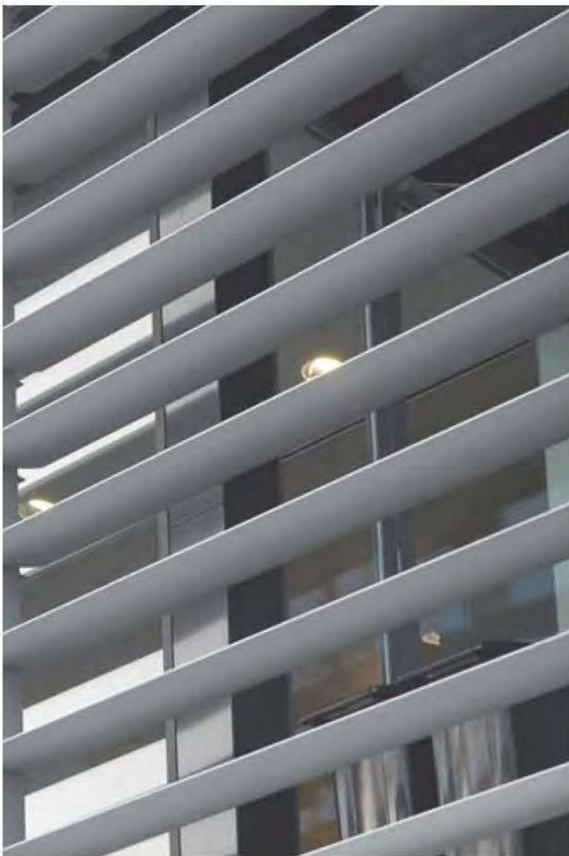
Anodised horizontal louvres to North facing homebases
