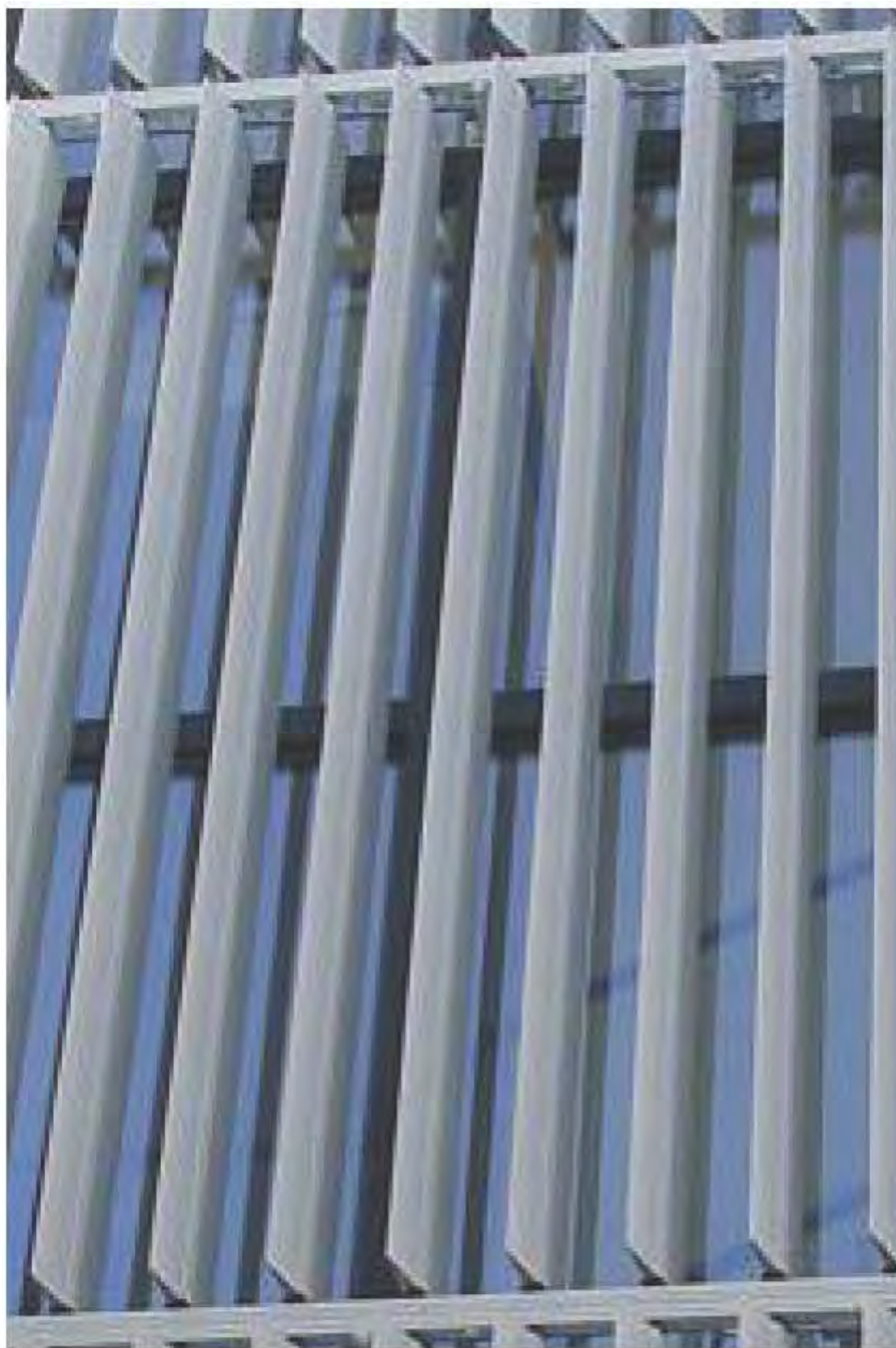
Anodised vertical louvres to South, East and West homebases
