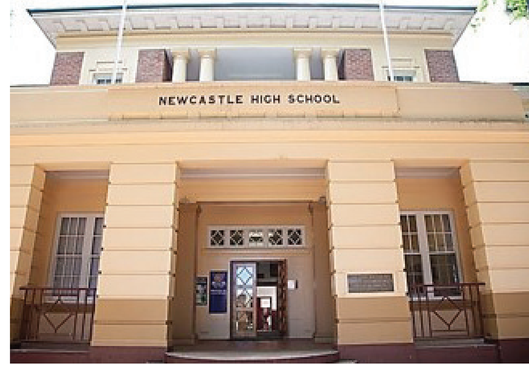
Building A entry
