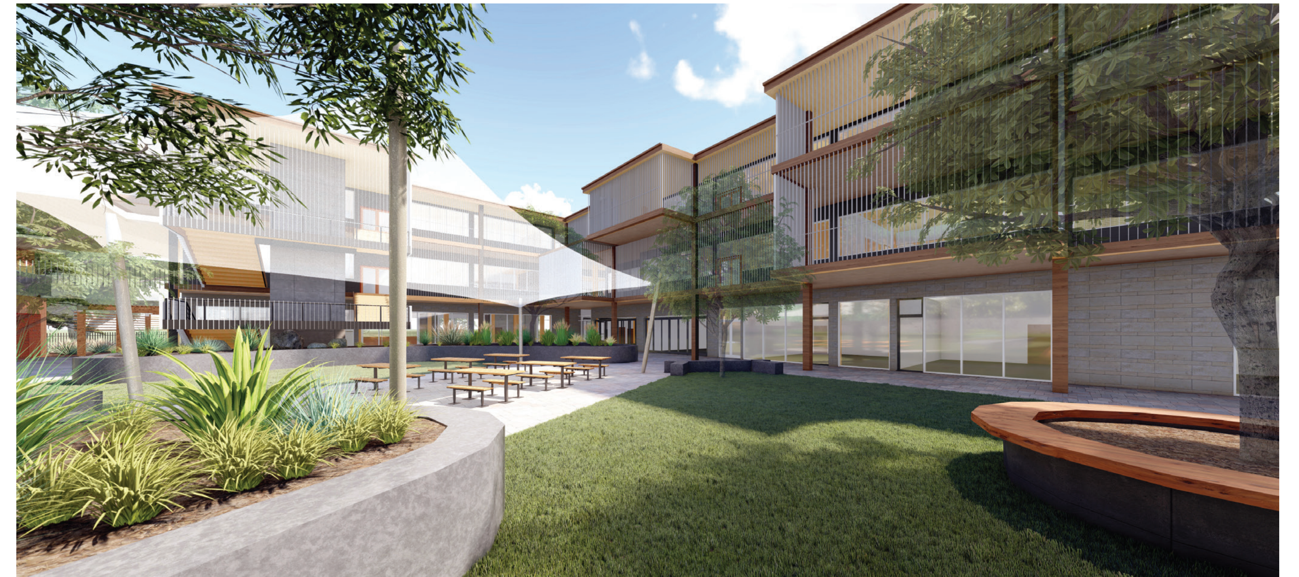
Internal courtyard of the new learning hub
