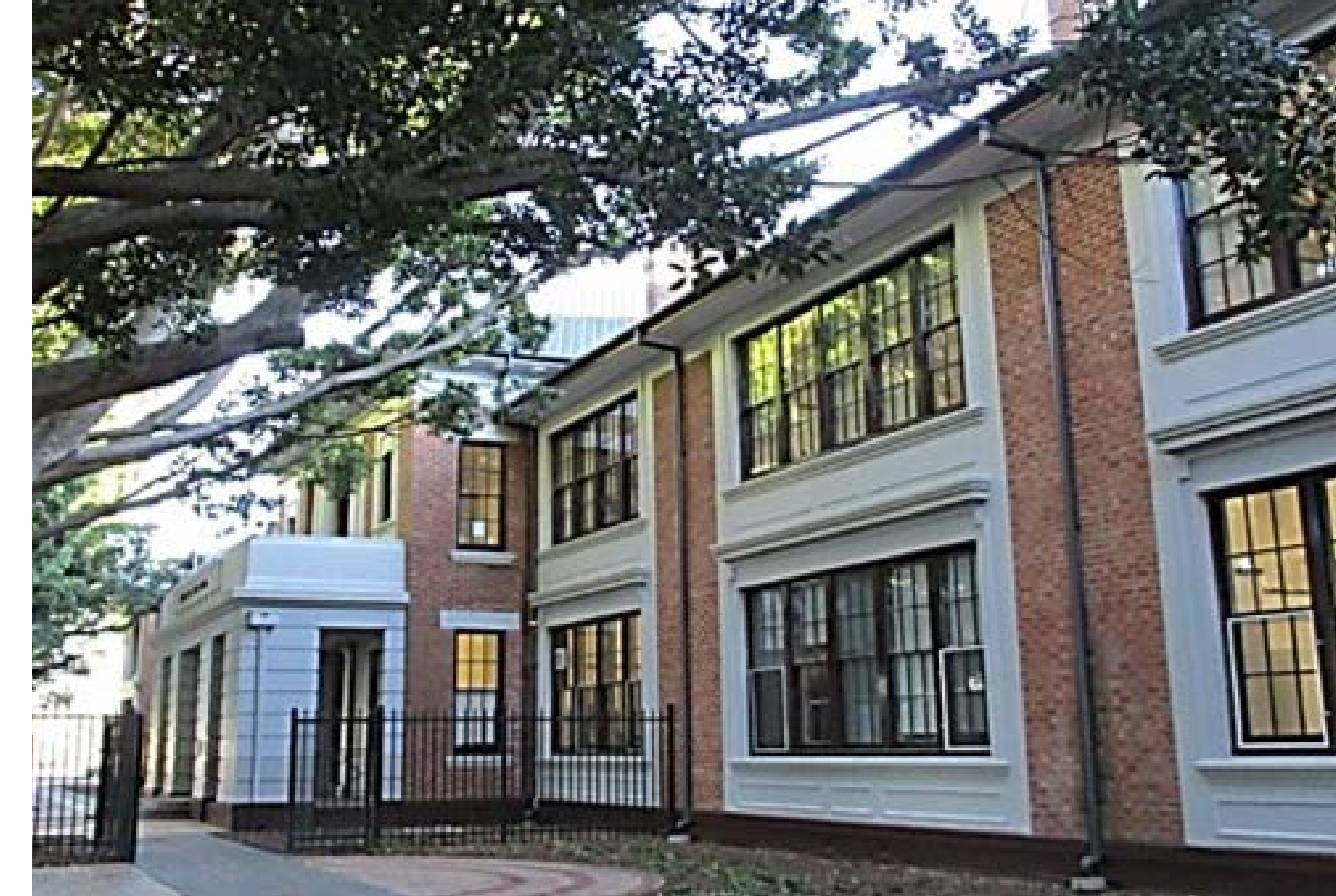
Building A administration
