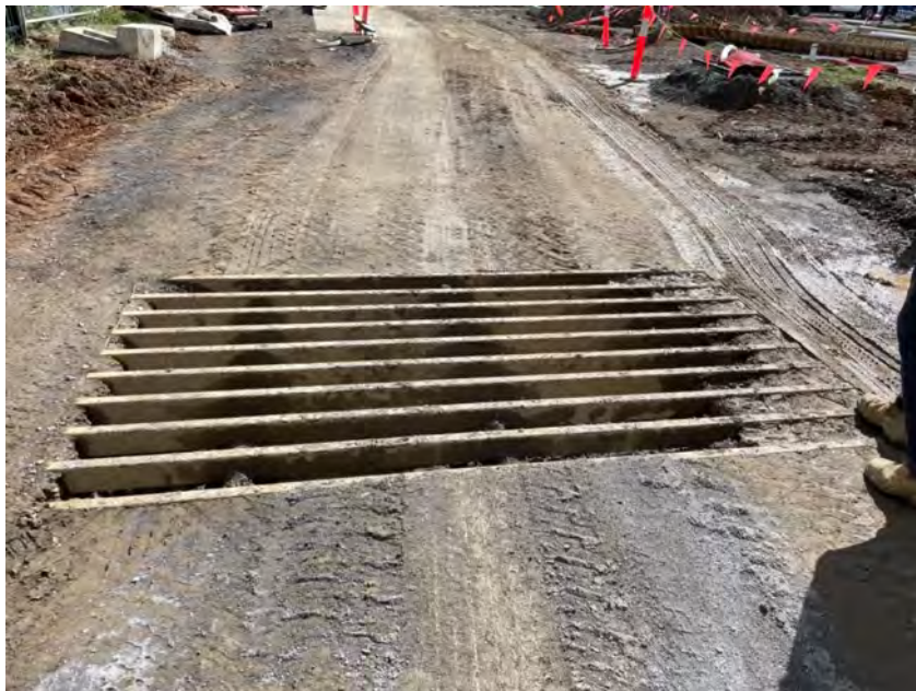
Photo 7 Entry/ exit point to site with rumble grid
