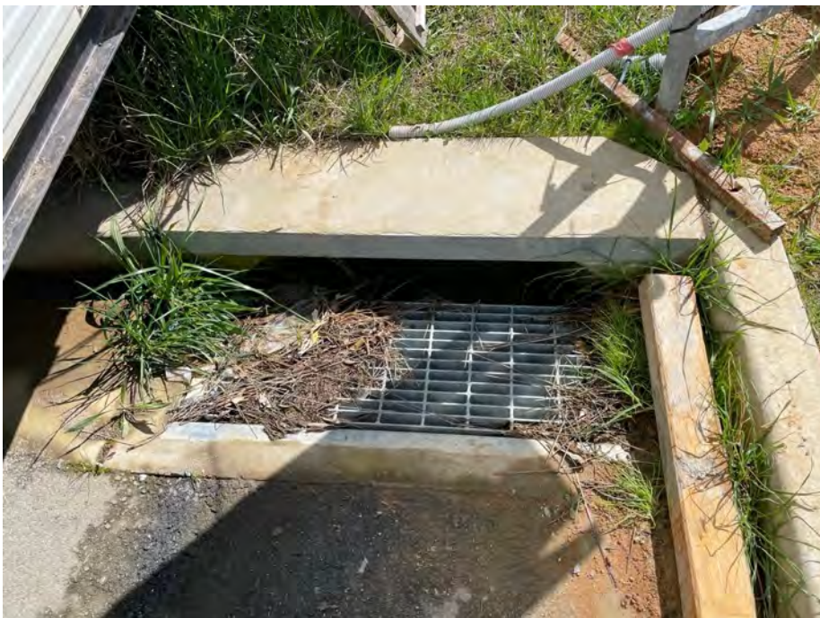
Photo 10 Unprotected stormwater drain behind site sheds
