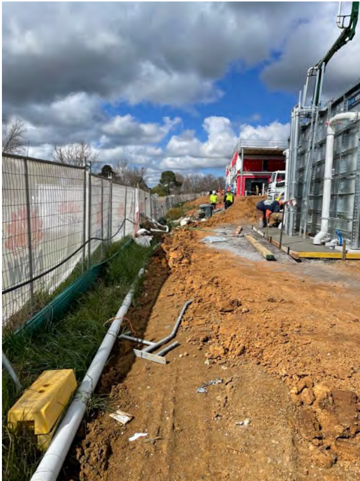
Photo 15 Sediment fencing along boundary
