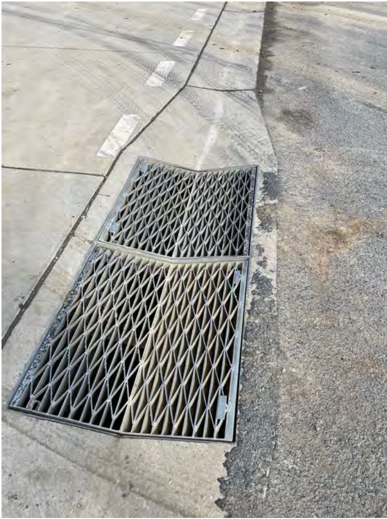
Photo 9 Unprotected stormwater drain at entry/exit to site
