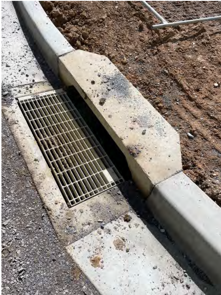
Photo 8 Unprotected stormwater drain at entry/exit to site
