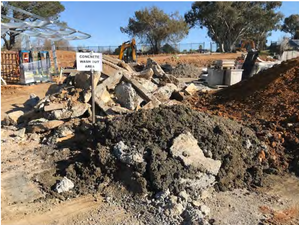
Photo 16 Designated concrete washout location
