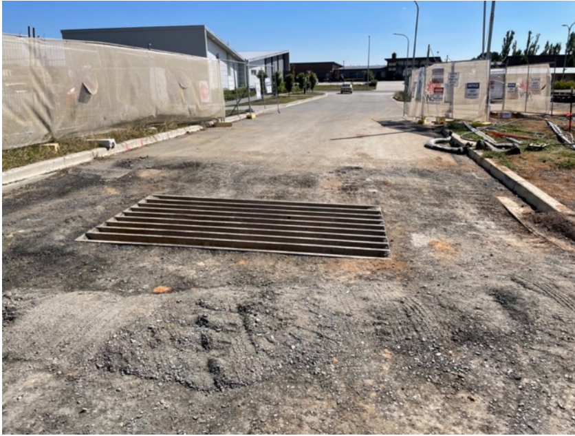
Photo 5 Entry/ exit point to site with rumble grid
