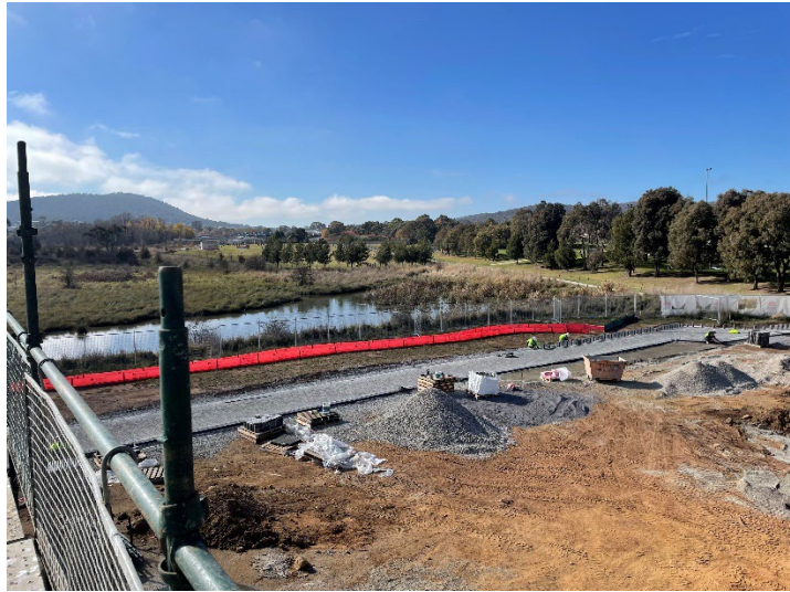
Newly installed erosion and sediment controls on boundary
