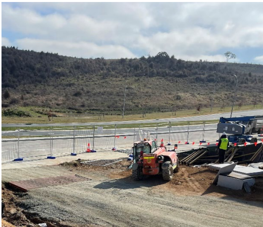
Rumble Grid at site exit
