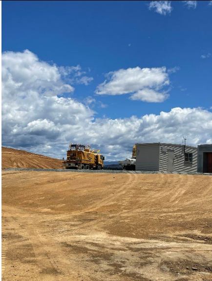
Compacted site to limit dust generation
