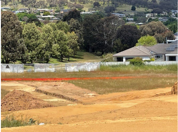
Site boundary showing fencing
