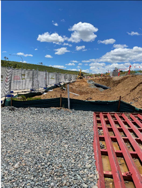
Rumble grids and rip rap at exits
