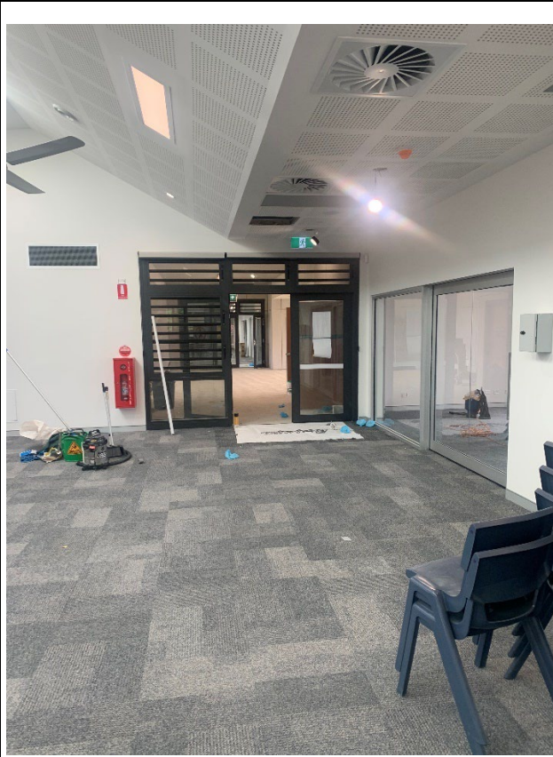
Egress between buildings
