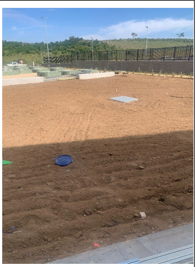
Ripped and topsoiled area
