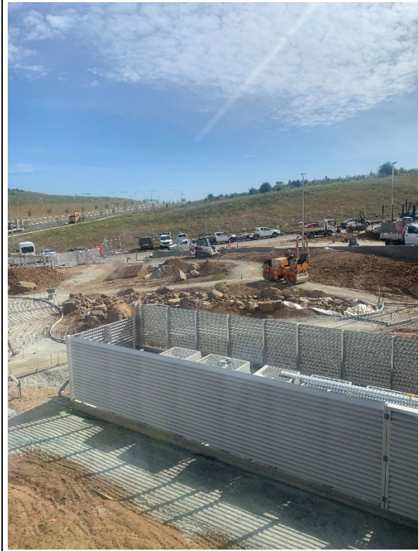
Landscaping works underway
