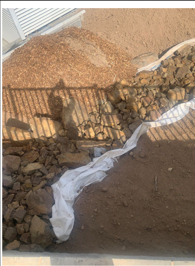
Rock lining swale drain
