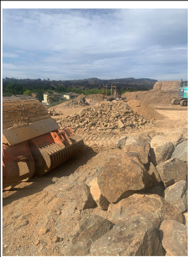
Remainder of earth/rock works for reinstatement
