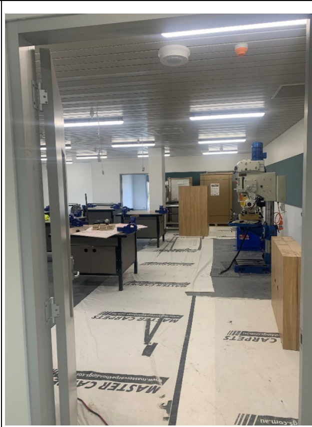
Near-completed classroom (manual arts)
