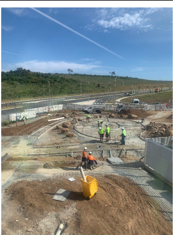
Landscaping (nature walking track) installation
