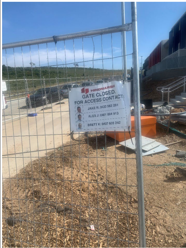
Security fencing preventing public access
