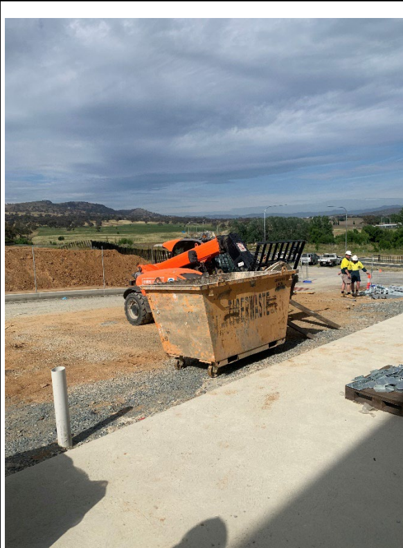
Waste receptacle (skip bin) serviced and clear
