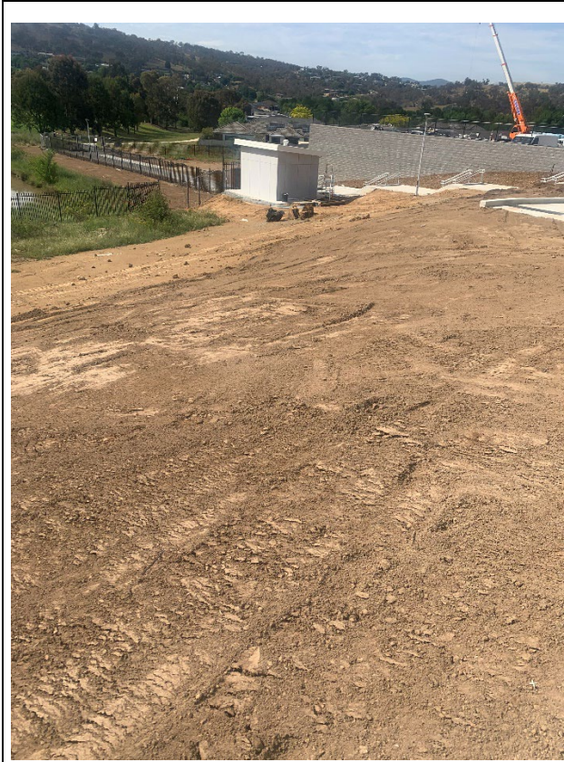
Vegetation buffer at bottom of slope as per ESCP
