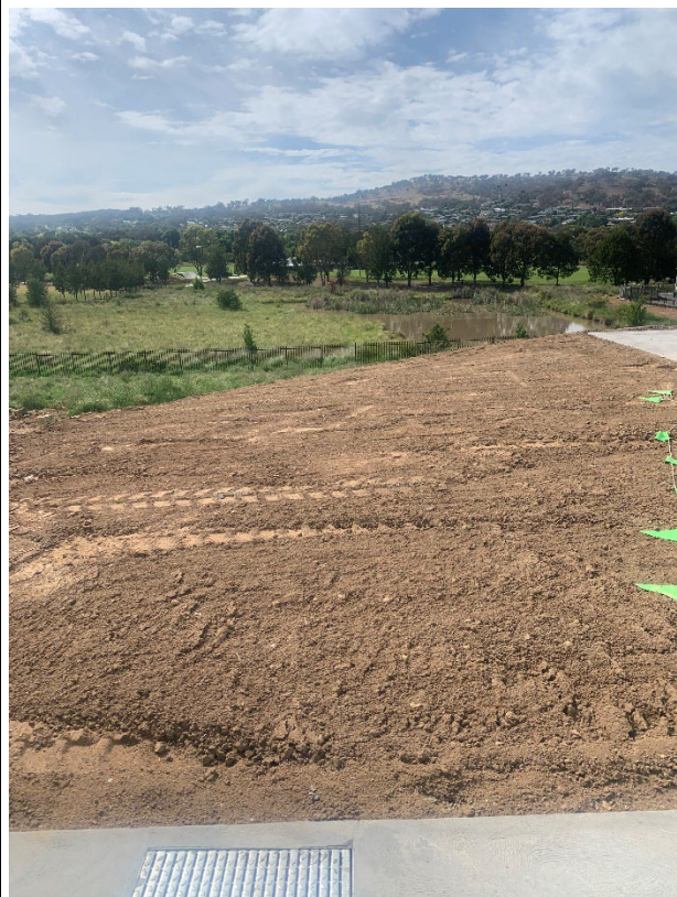
Remaining exposed areas (lightly compacted)
