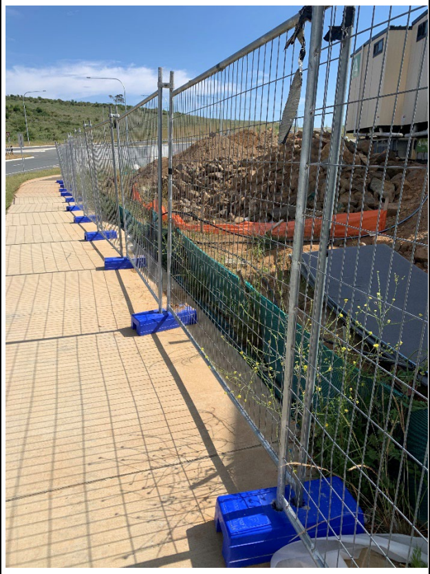
Security fencing preventing public access
