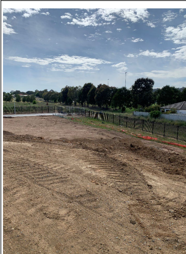
Remaining exposed areas, vegetated buffer in tact
