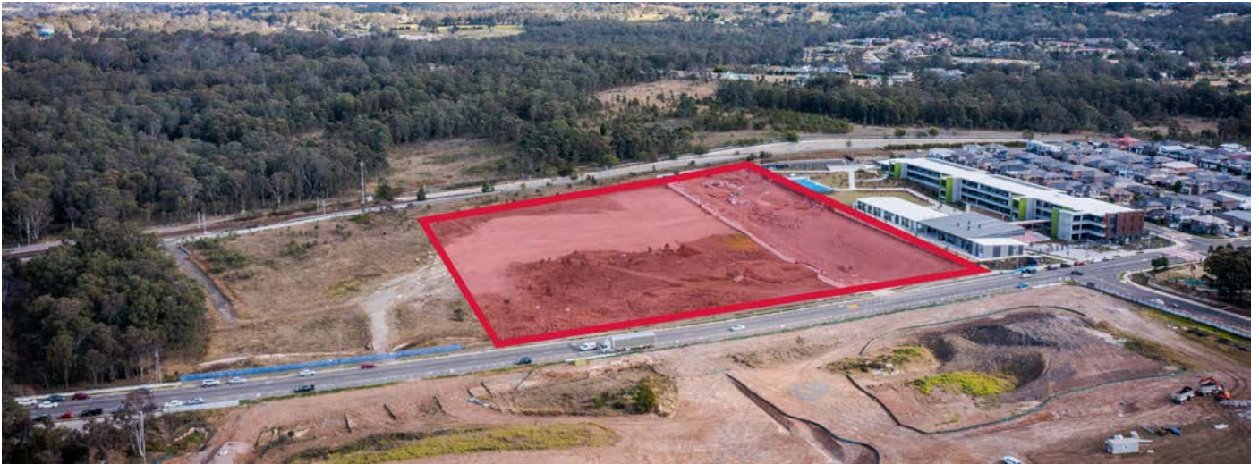
Site location next to the Edmondson Park Public School on Buchan Avenue, Edmondson Park
