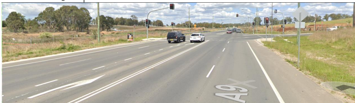
Figure 31 - The Northern Road – Southbound towards Bradley Street
