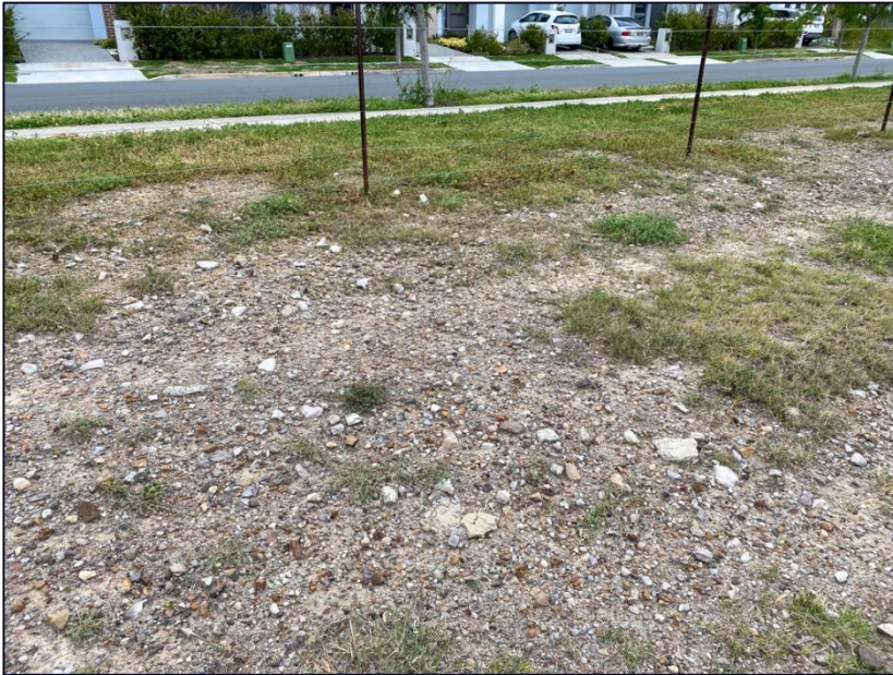
Photograph 3: Area along raised southern boundary with exposed rubble and clay fill
