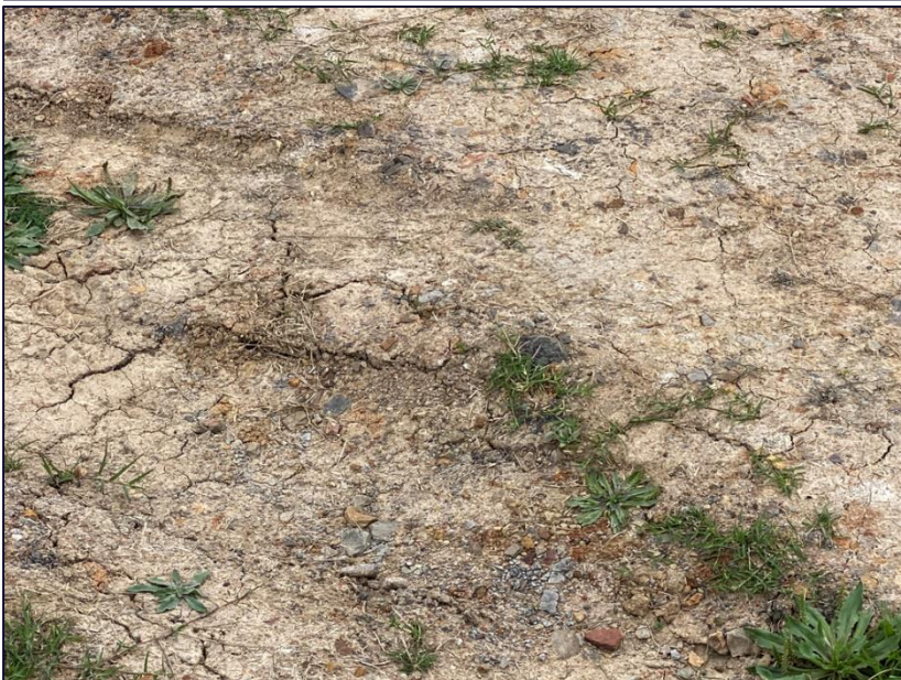
Photograph 2: Exposed area revealing redeposited clay fill
