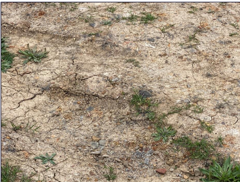
Photograph 2: Exposed area revealing redeposited clay fill
