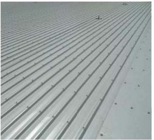
CORRUGATED METAL ROOF 'SHALE GREY'
