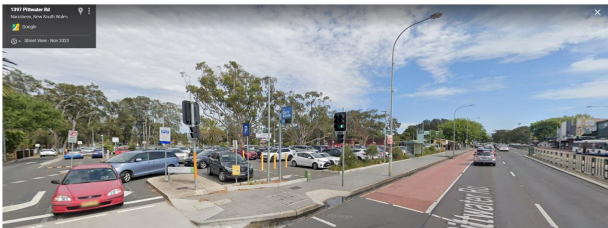
Figure 24: Narrabeen B1 Bus Car Park
