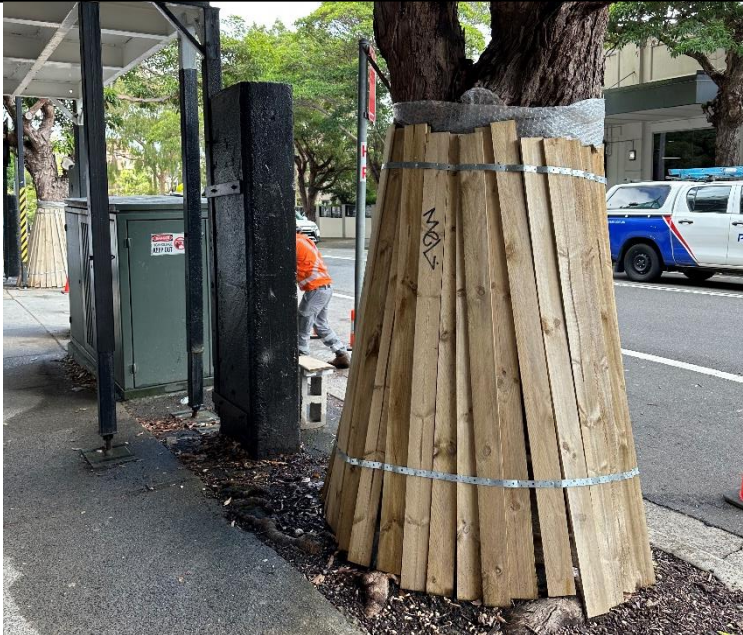
PHOTOGRAPH 11: TREE PROTECTION MEASURES
