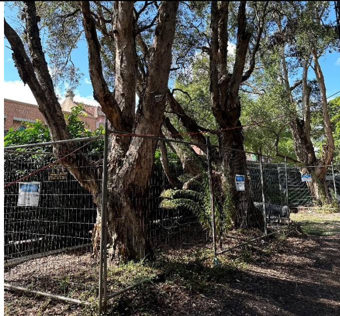
PHOTOGRAPH 12: TREE PROTECTION MEASURES
