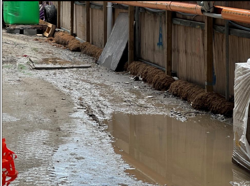
PHOTOGRAPH 4: SEDIMENT AND EROSION CONTROLS AT CONSTRUCTION ZONE BOUNDARY
