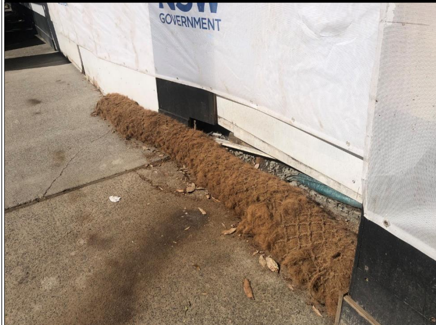
PHOTOGRAPH 4: SEDIMENT AND EROSION CONTROLS AT SITE BOUNDARY
