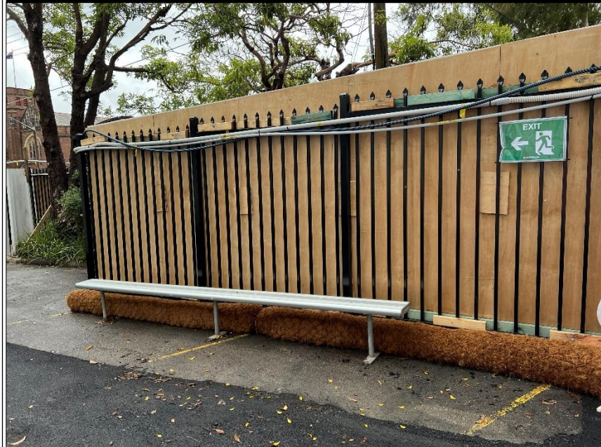
PHOTOGRAPH 4: SEDIMENT AND EROSION CONTROLS AT SITE BOUNDARY
