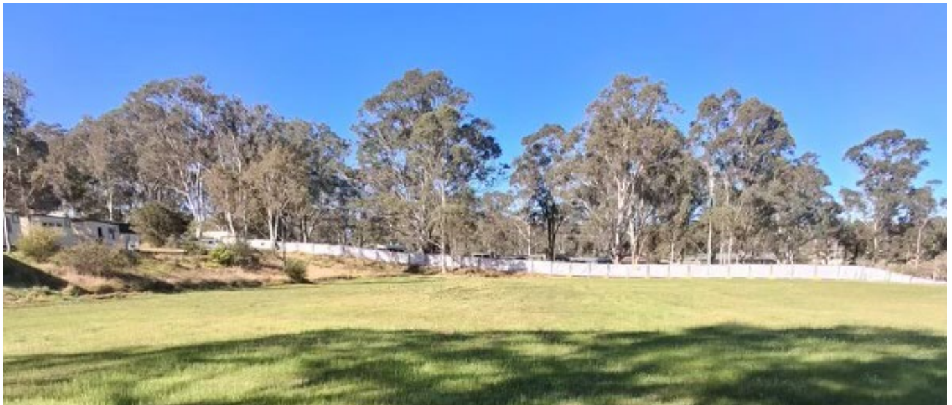
The construction compound at Moruya High School
