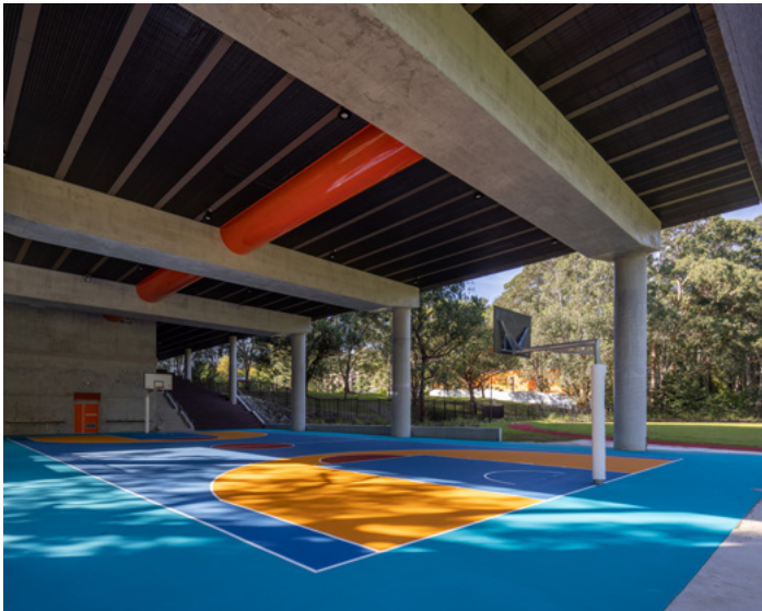
Example of a covered outdoor learning area (COLA)
