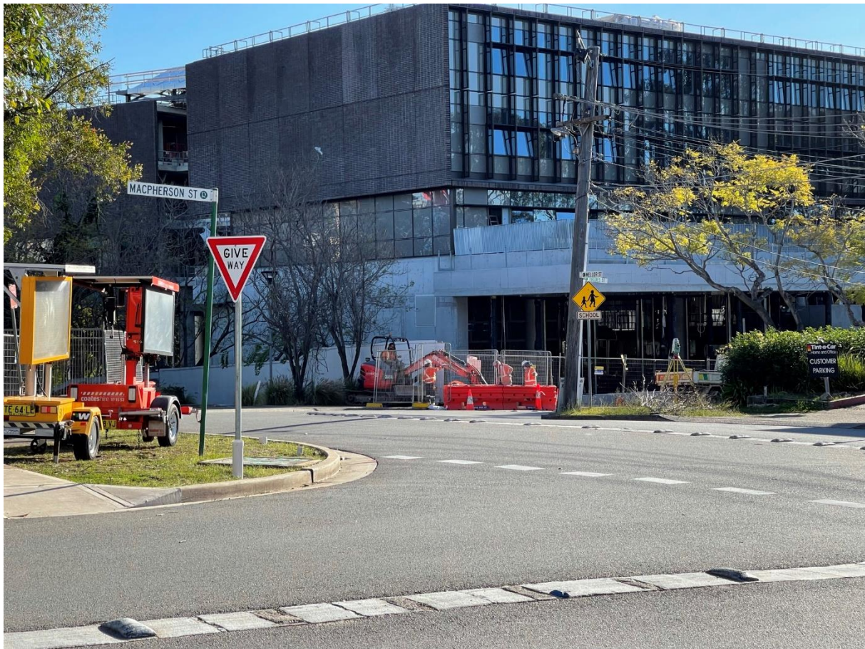
Figure 3 Rhodes Street Civil Works TAFE NSW site- Driveway
