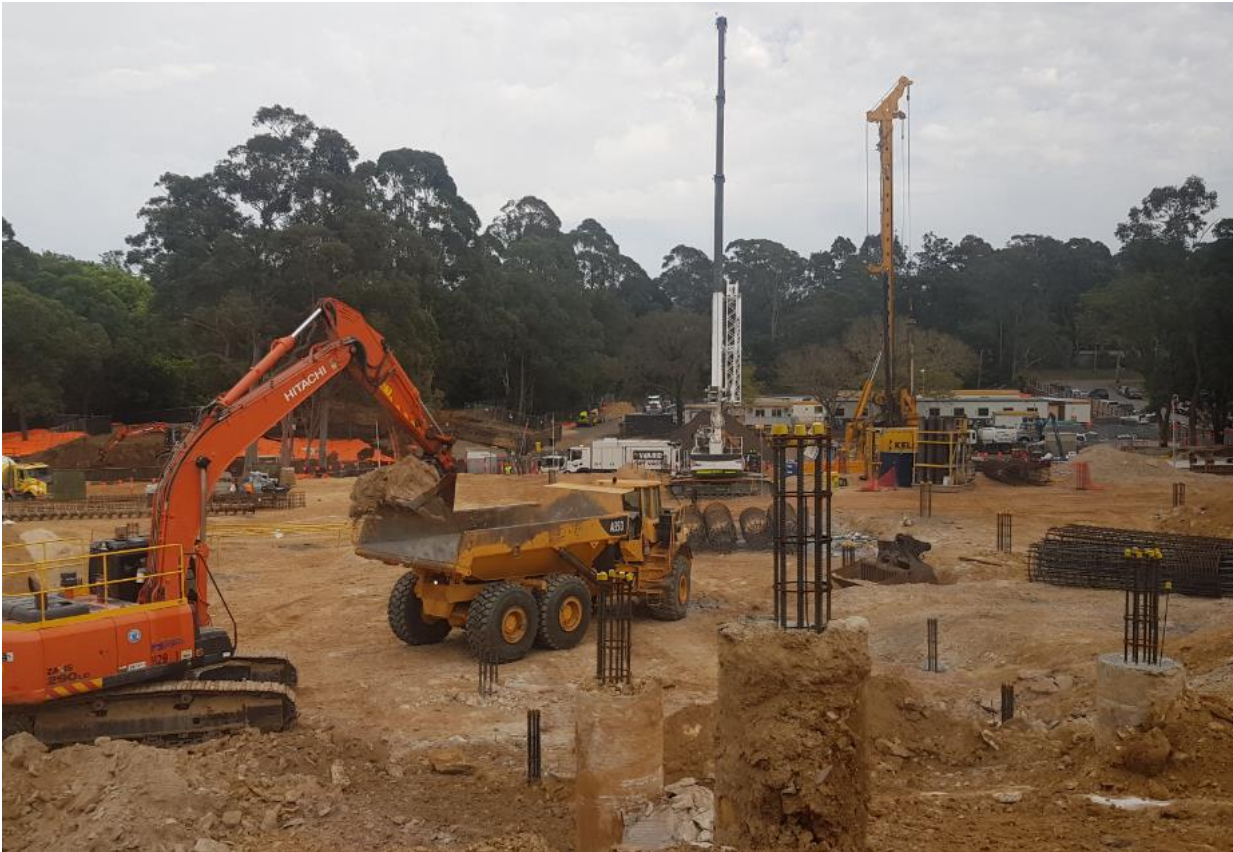
Photo 8: Earthworks and piling in process.
