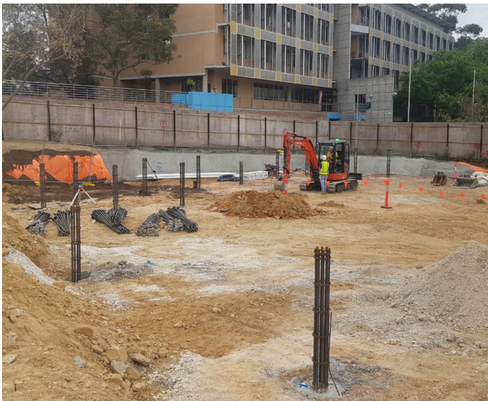
Photo 6: Piles installed with the existing TAFE in the background
