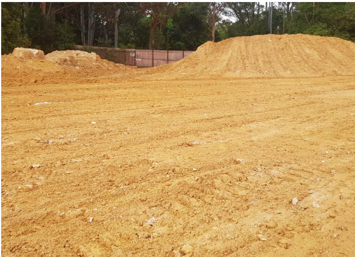
Photo 4: Spreading and compaction of imported VENM.
