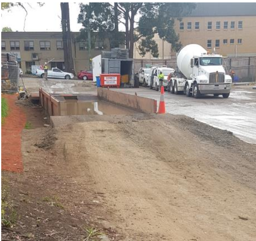
Photo 7: Wheel wash in place
