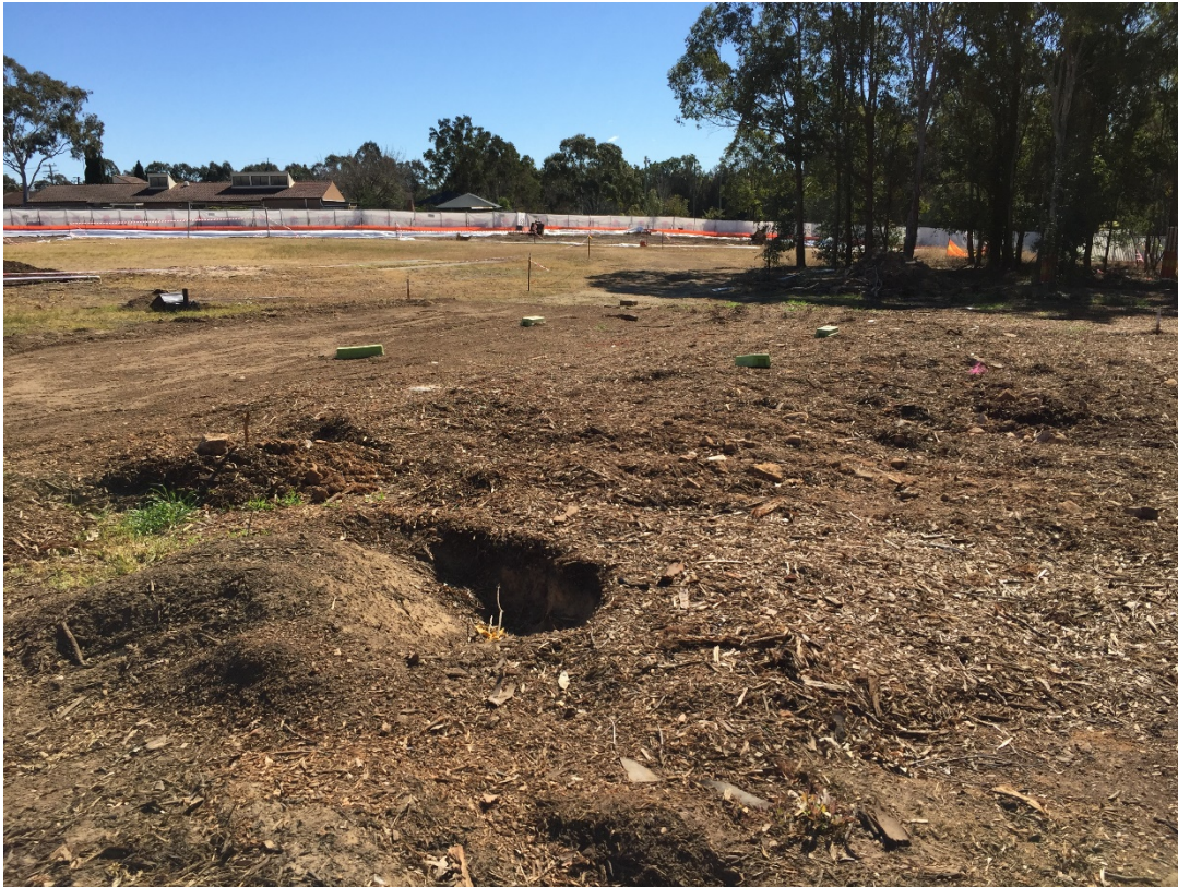
Photo 9: This shows some of the mulch material that has been used for dust and erosion suppression over part of the western section of the Site
