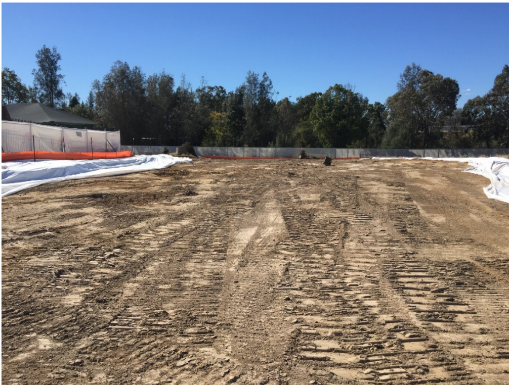
Photo 12: View looking east over the northern section of Area 1. Note the geofabric covering the edges of the excavation and the sediment fencing
