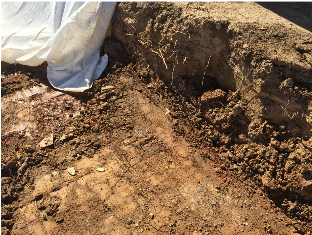
Photo 14: This cutting is located along the western Site boundary in Area 4. Evidence of what appeared to be fragments of asbestos cement sheeting were observed on the surface and in the cutting. The cutting was kept covered
