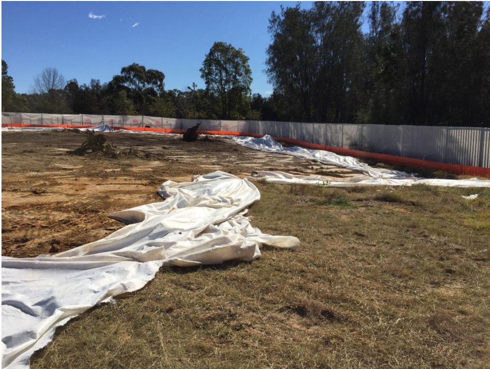
Photo 11: View looking north to the northern corner of the Site and the eastern section of Area 1. Note the geofabric covering the edges of the excavation and the sediment fencing
