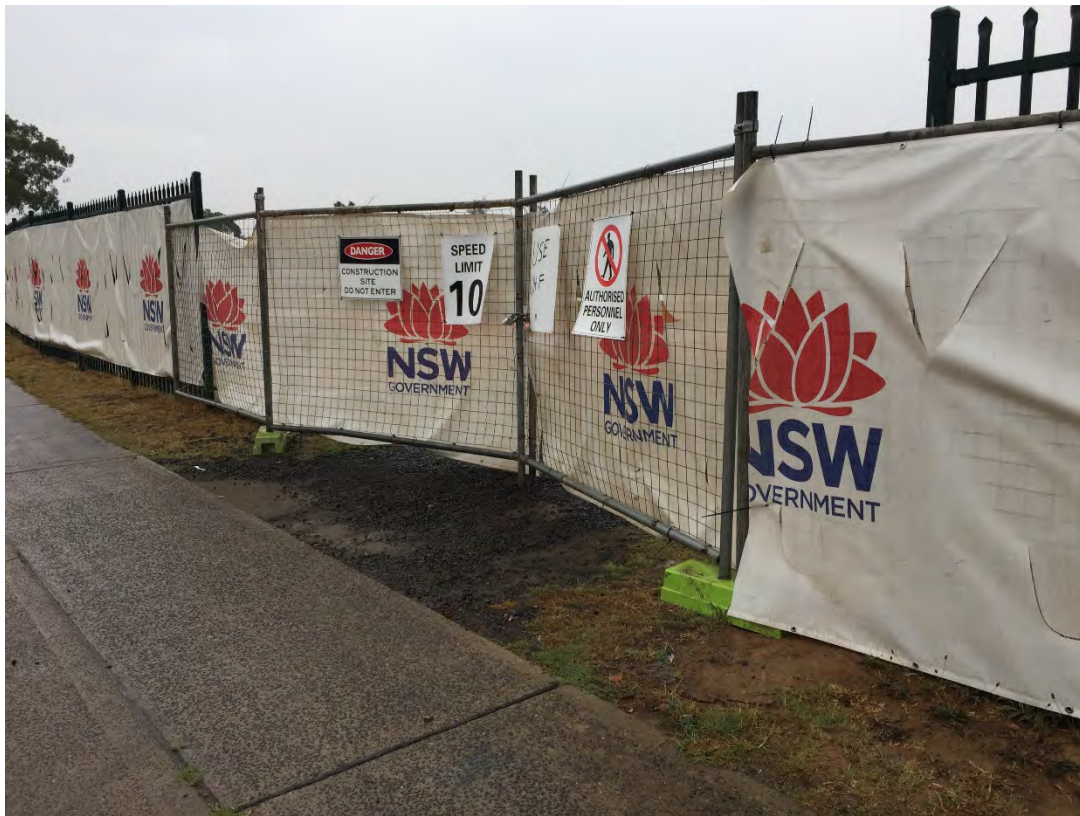
Photo 13: Temporary construction site gate with signage
