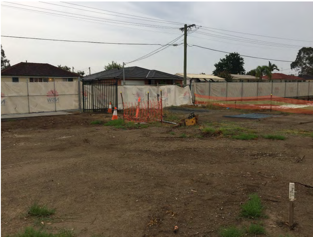
Photo 2: View of the site entry gate to the site
