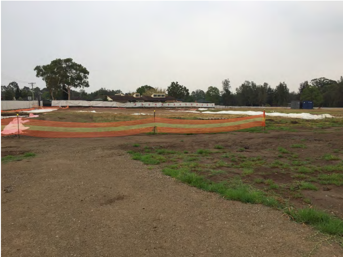
Photo 3: View looking north across the site from near the site compound
