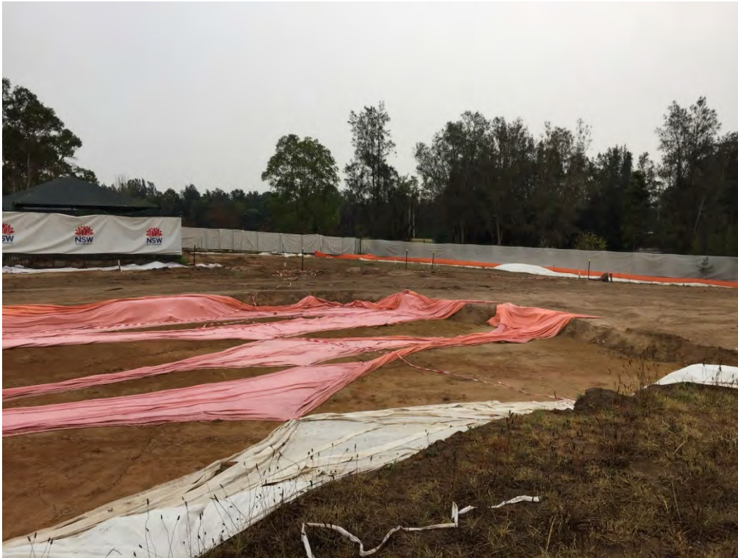
Photo 9: View over the northeast corner of the site. Some of the lining used to cover exposed soils needed to be reinstated
