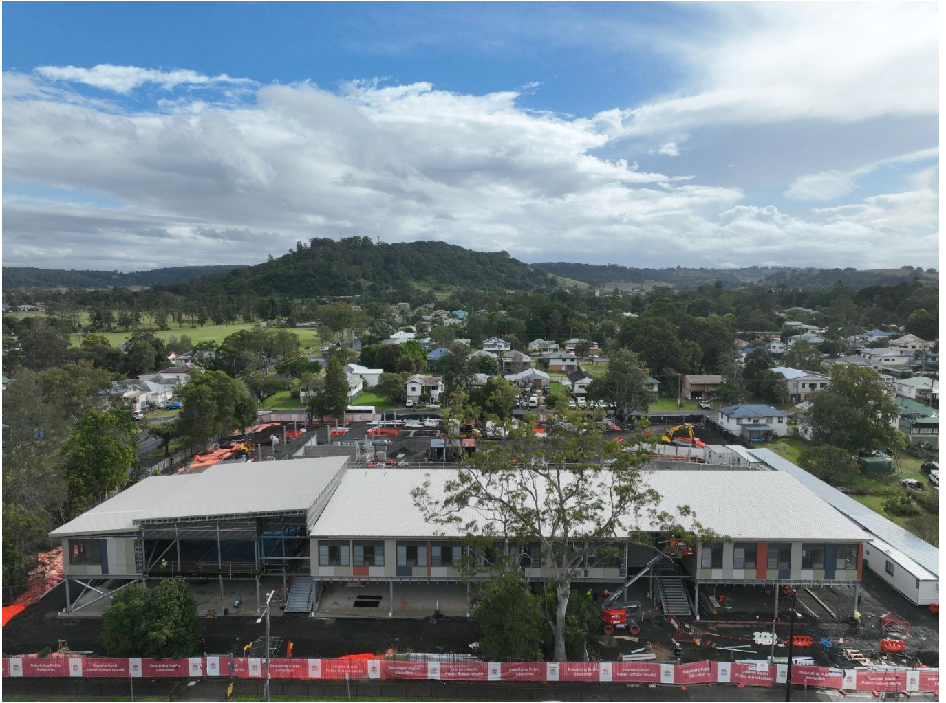
Lismore South Public School taking shape along Kyogle Street.
