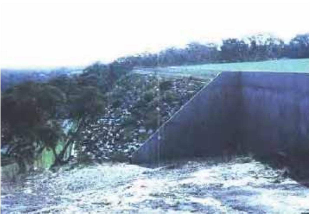
Figure 219 – Battered slope and natural rock retaining wall to Oval, with concrete wall for future Gymnasium
