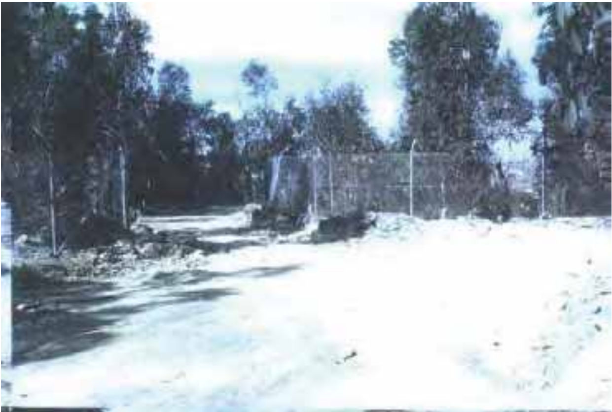
Figure 218 – Careful protection placed around natural landscape during construction works
