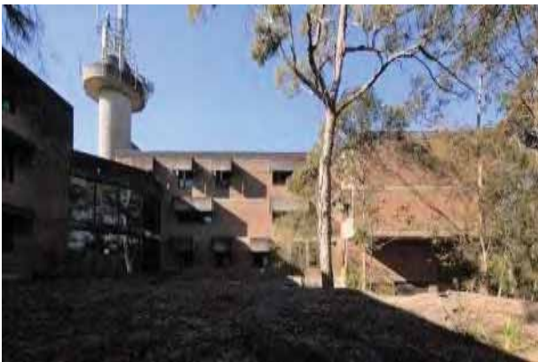
Figure 39 – Portion of western elevation, featuring pre-cast concrete window hoods
