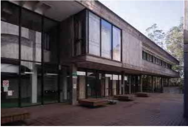
Figure 93 – Southern elevation adjacent to courtyard (bound to the south by Stage 1), featuring off-board concrete
