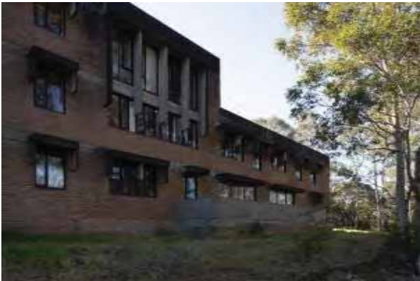
Figure 43 – Portion of southern elevation, with face brickwork and pre-cast concrete sunshades and window hoods
