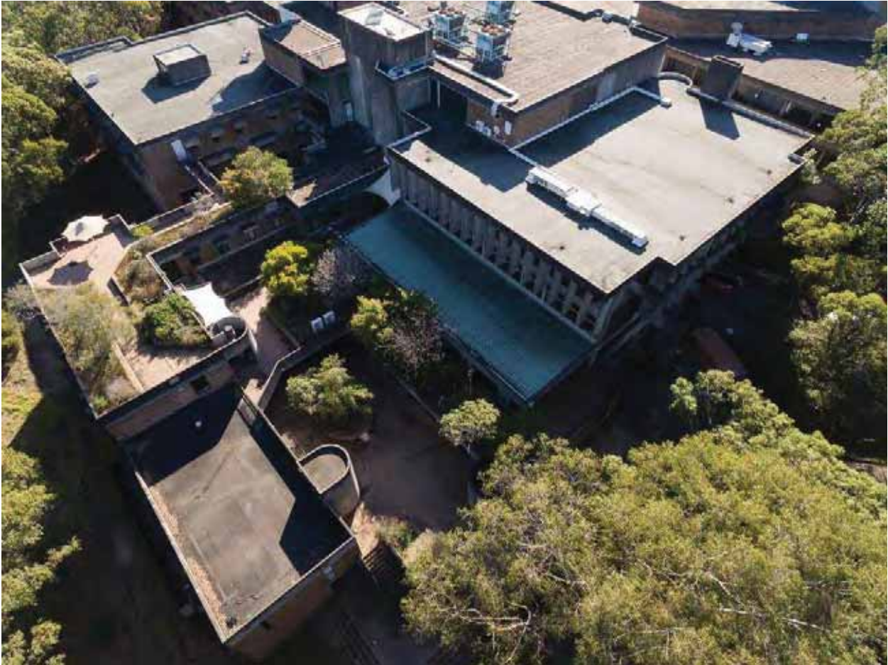
Figure 38 – Oblique aerial view showing the south-eastern portion of Stage 1 building, with extensive use of off-board concrete and face brickwork, integrated with rooftop gardens and courtyards.
