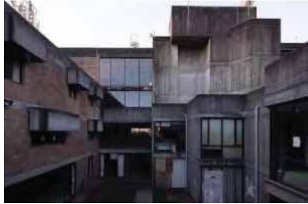
Figure 42 – Portion of southern elevation, with massing of off-board concrete forms and pre-cast concrete window hoods
