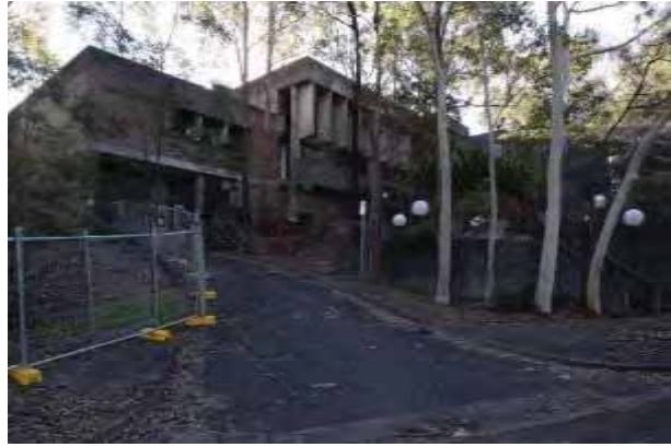
Figure 94 – Portion of Eastern elevation featuring pre-cast concrete sunshades
