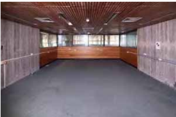
Figure 57 – Space within former library located on Level 5 showing the distinctive battened ceiling and off board concrete walls
