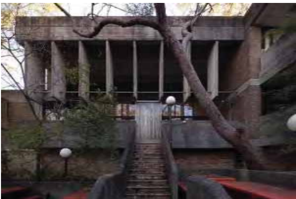
Figure 91 – Section of eastern elevation (outside cafeteria space) featuring pre-cast concrete sunshade
