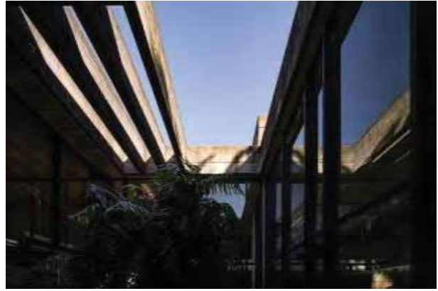
Figure 126 – Atrium at Levels 5 with pre-cast concrete fins spanning across the pond/ open space. Source: Alexander Mayes
