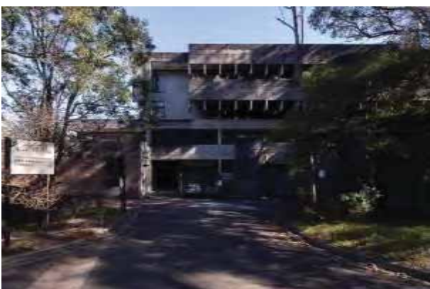
Figure 45 – Portion of eastern elevation with large sections of off-board concrete and sunshades
