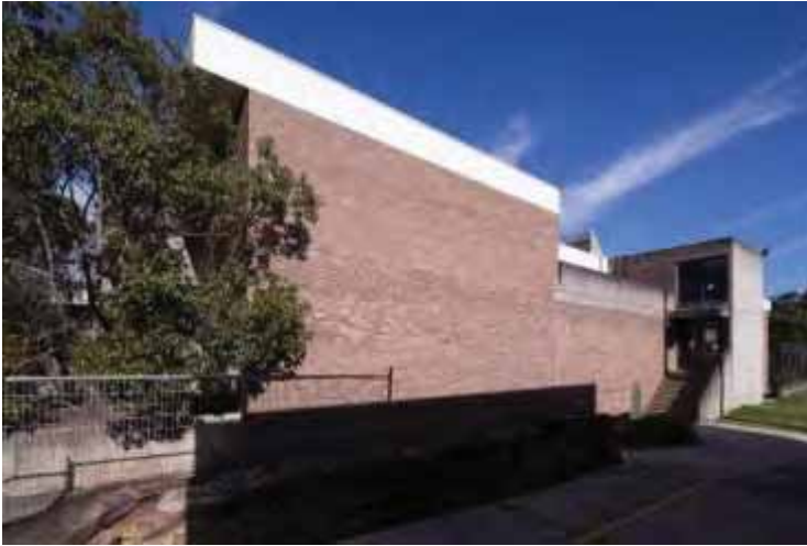
Figure 134 – Northern elevation of the Stage 3 building set on natural sandstone base, with facebrick walls
