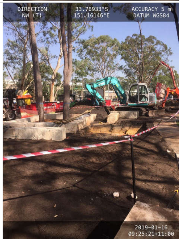
Photograph 6: Taken showing the remediation area where asbestos cement fragments were identified, facing north-west. Note the excavated area and the imported topsoil in the immediate vicinity.
