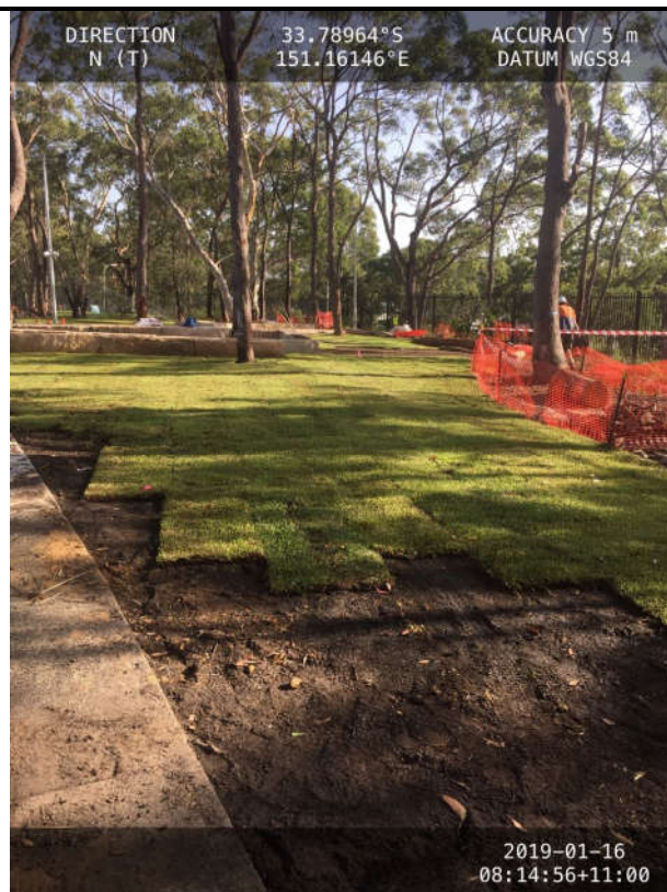
Photograph 1: Taken showing part of the eastern portion of the site, facing north. Note the dense recently laid grass turf covering the ground and imported topsoil beneath.
