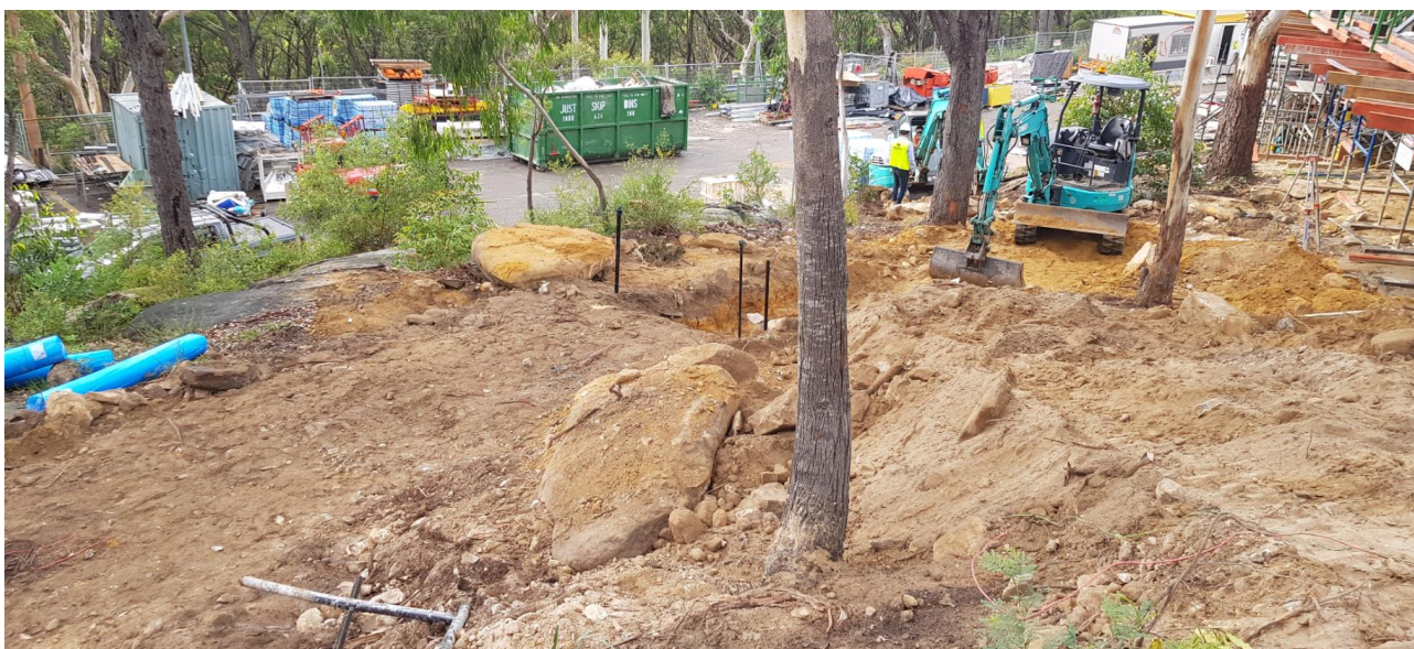
Photo 4: Excavation within tree protection zones without arborist supervision
