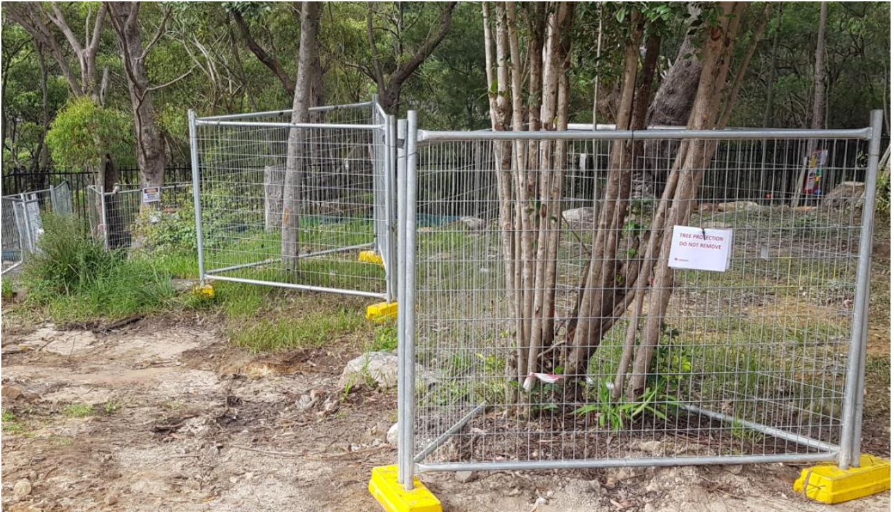
Photo 8: Tree protection zones in place
