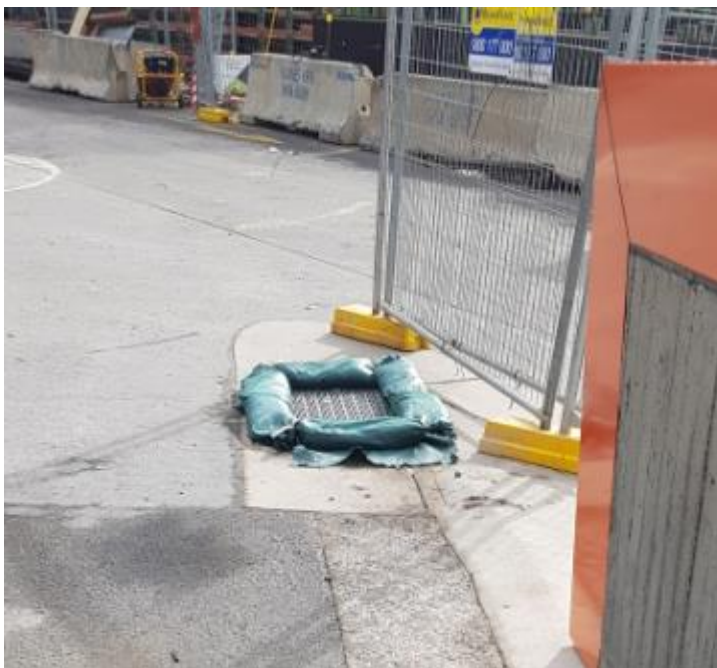
Photo 3: Drain protection
