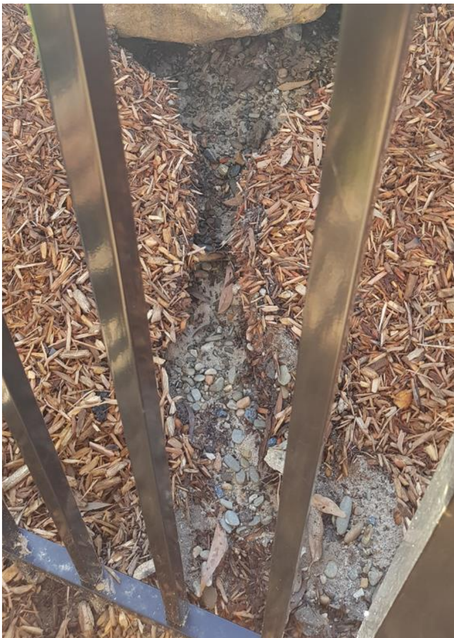
Photo 11: Evidence of scouring / high velocity flow leaving the site from on site detention basin. Remedial work required.
