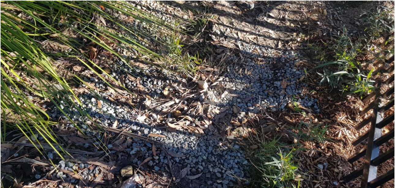
Photo 10: Evidence of high velocity flow leaving the site and entering the Lane Cove National Park. Remedial work required.
