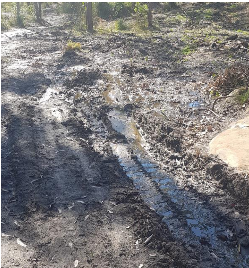
Photo 9: Dunstan Grove APZ with insufficient ground cover. Remedial work required.
