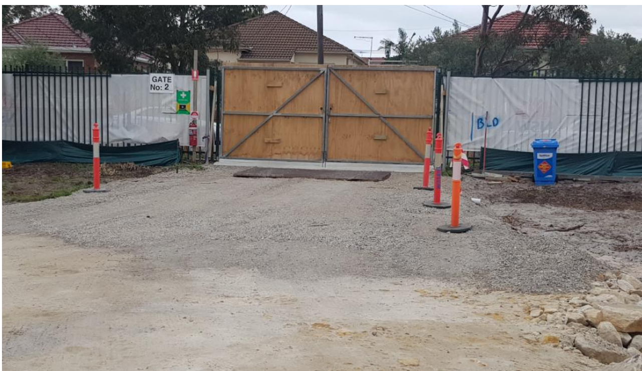
Photo 4: Stabilised site access.
