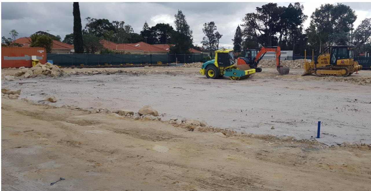
Photo 3: Site establishment. Note haul road compacted and 10T roller in shot.
