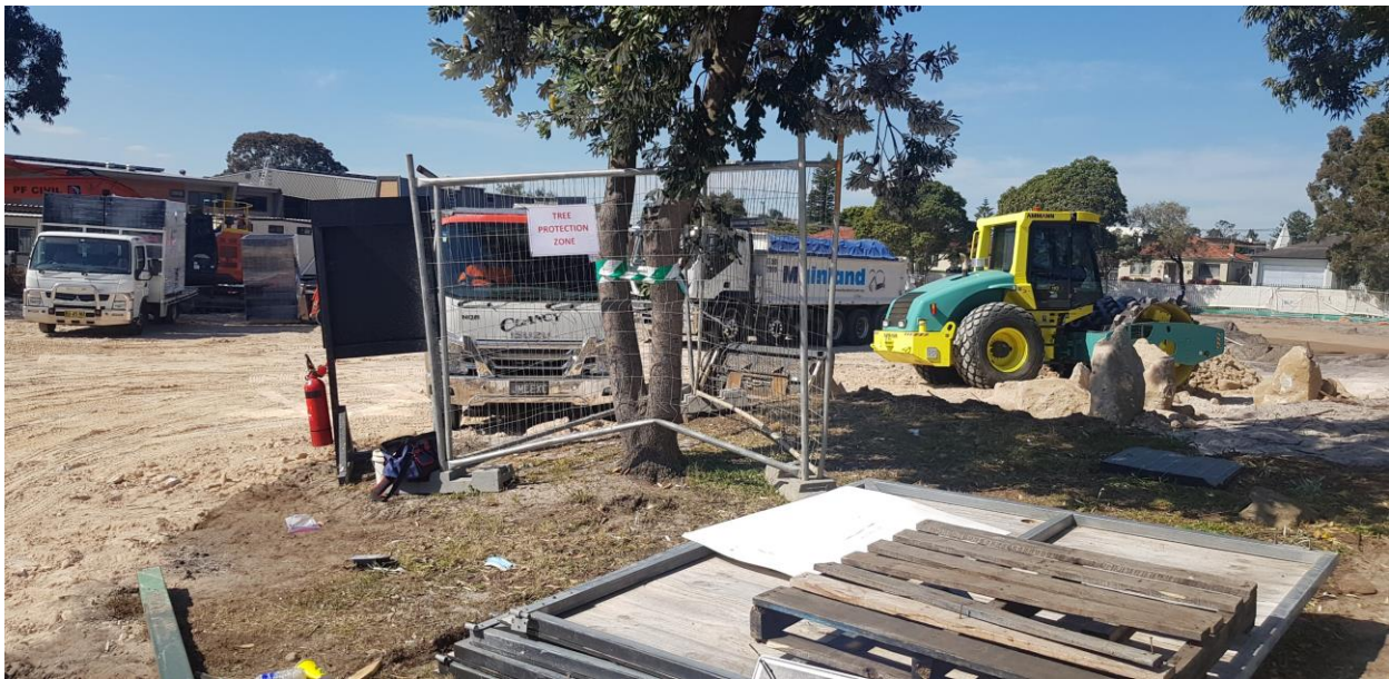
Photo 3: Tree Protection Zone, site inspection (19/08/21).
