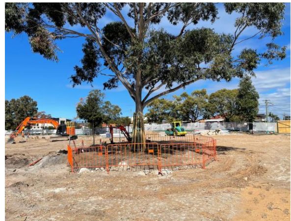
Photo 2a: Tree Protection Zone during site inspection (19/08/21) and 2b evidence of improvement during virtual audit (26/08/21)
