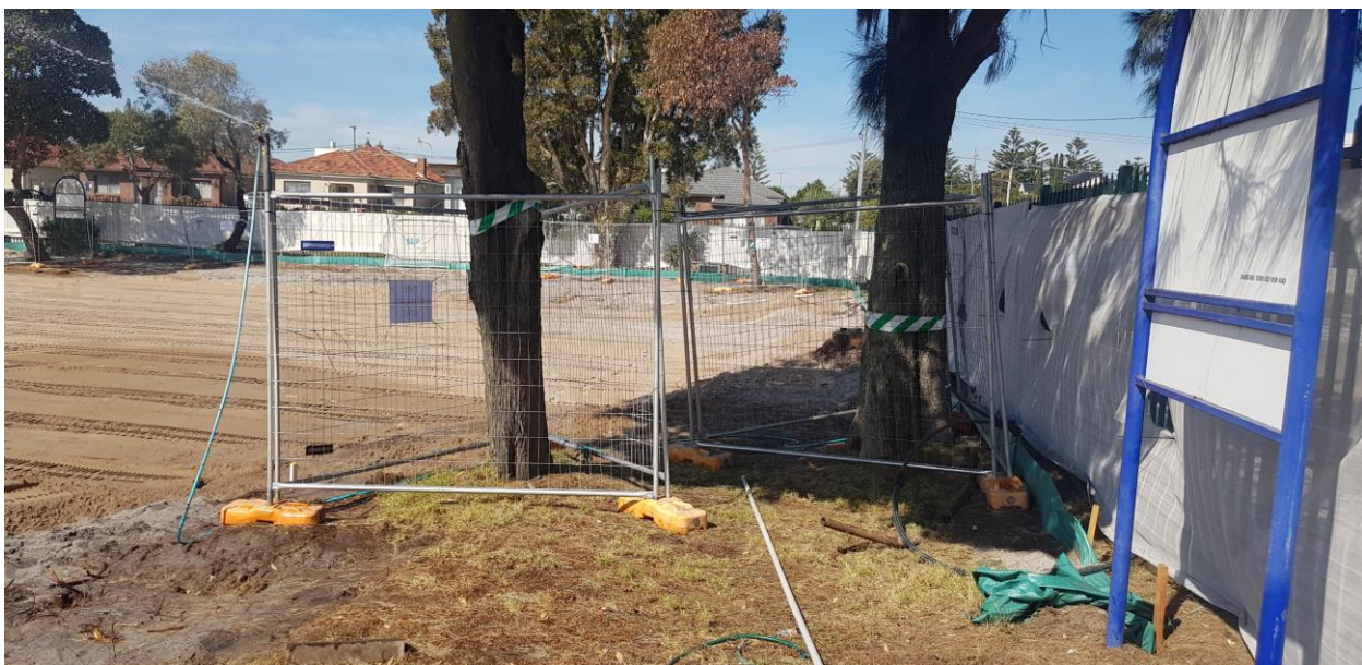
Photo 4: Tree Protection Zone, site inspection (19/08/21).
