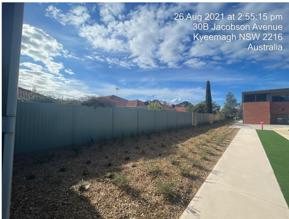
Photo 8: Acoustic barrier located on the north-west boundary
