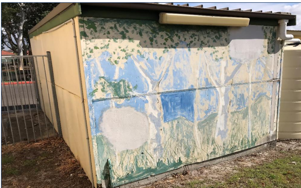
Photograph 4: Clad buildings adjacent to Jacobson Avenue with potential ACM wall linings.
