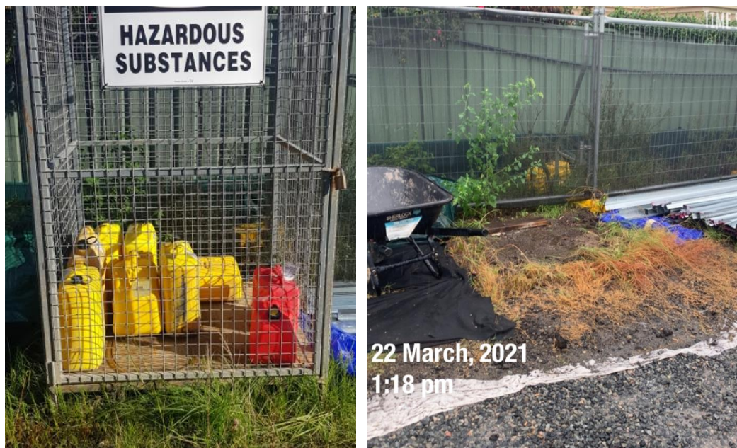
Photo 1a and 1b: Un-bunded fuel storage (left) and removed from site (right)
