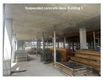
Current work is focussed on Building 1. Ground floor and level 1 suspended slabs have been poured for Building 1, together with most of the columns to the roof. Final pouring of columns should be completed late March 2024.
