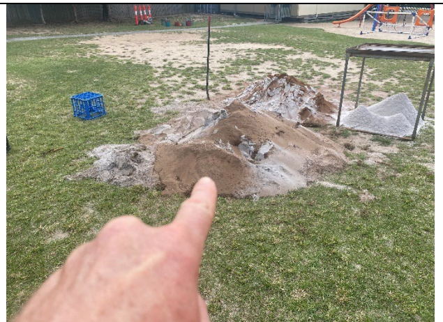
Photo 2: Stockpiled material excavated from trench
