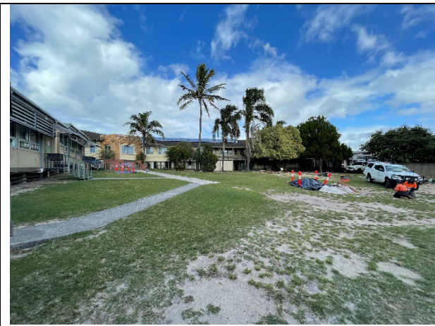
Photo 1: Site location with trench and stockpiles in background
