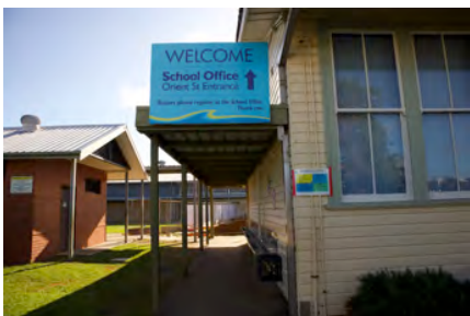
Photo #: IMG0142.jpg Caption: External - West along southern side of CR0030 Camera Model: Canon EOS M50 Focal Length: 15.00mm Shutter Speed: 1/320
