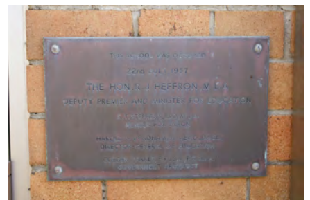
Photo #: IMG0132.jpg Caption: External - Plaque #1 detail left of entrance to CR0012 Camera Model: Canon EOS M50 Focal Length: 37.00mm Shutter Speed: 1/80
