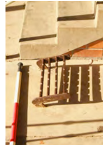
Photo #: IMG0105.jpg Caption: External - Detail of Boot Scrubber at bottom of stairs to CR0034 Camera Model: Canon EOS M50 Focal Length: 45.00mm Shutter Speed: 1/160
