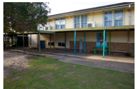
Photo #: IMG0108.jpg Caption: External - North towards CR0004 & CR0006 Camera Model: Canon EOS M50 Focal Length: 17.00mm Shutter Speed: 1/160
