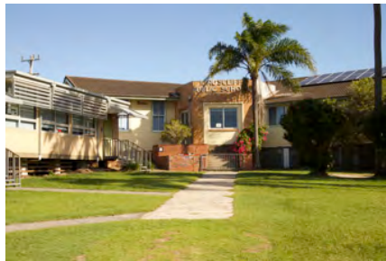
Photo #: IMG0125.jpg Caption: External - South towards CR0012 Camera Model: Canon EOS M50 Focal Length: 29.00mm Shutter Speed: 1/250
