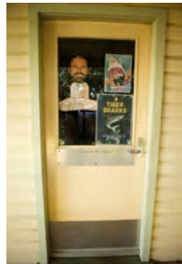
Photo #: IMG0155.jpg Caption: External - South from CR0007 towards door to CR0003 Camera Model: Canon EOS M50 Focal Length: 15.00mm Shutter Speed: 1/25
