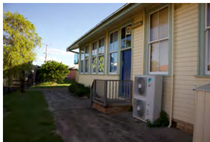
Photo #: IMG0140.jpg Caption: External - South along eastern side of CR0030 Camera Model: Canon EOS M50 Focal Length: 15.00mm Shutter Speed: 1/250
