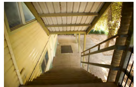
Photo #: IMG0153.jpg Caption: External - North west down stairs CR0035 Camera Model: Canon EOS M50 Focal Length: 15.00mm Shutter Speed: 1/30
