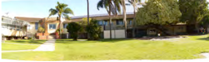
Photo #: IMG0121.jpg Caption: External - South towards CR0003 Camera Model: Canon EOS M50 Focal Length: 29.00mm Shutter Speed: 1/160
