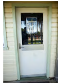
Photo #: IMG0156.jpg Caption: External - South from CR0007 towards door to CR0008 Camera Model: Canon EOS M50 Focal Length: 15.00mm Shutter Speed: 1/80
