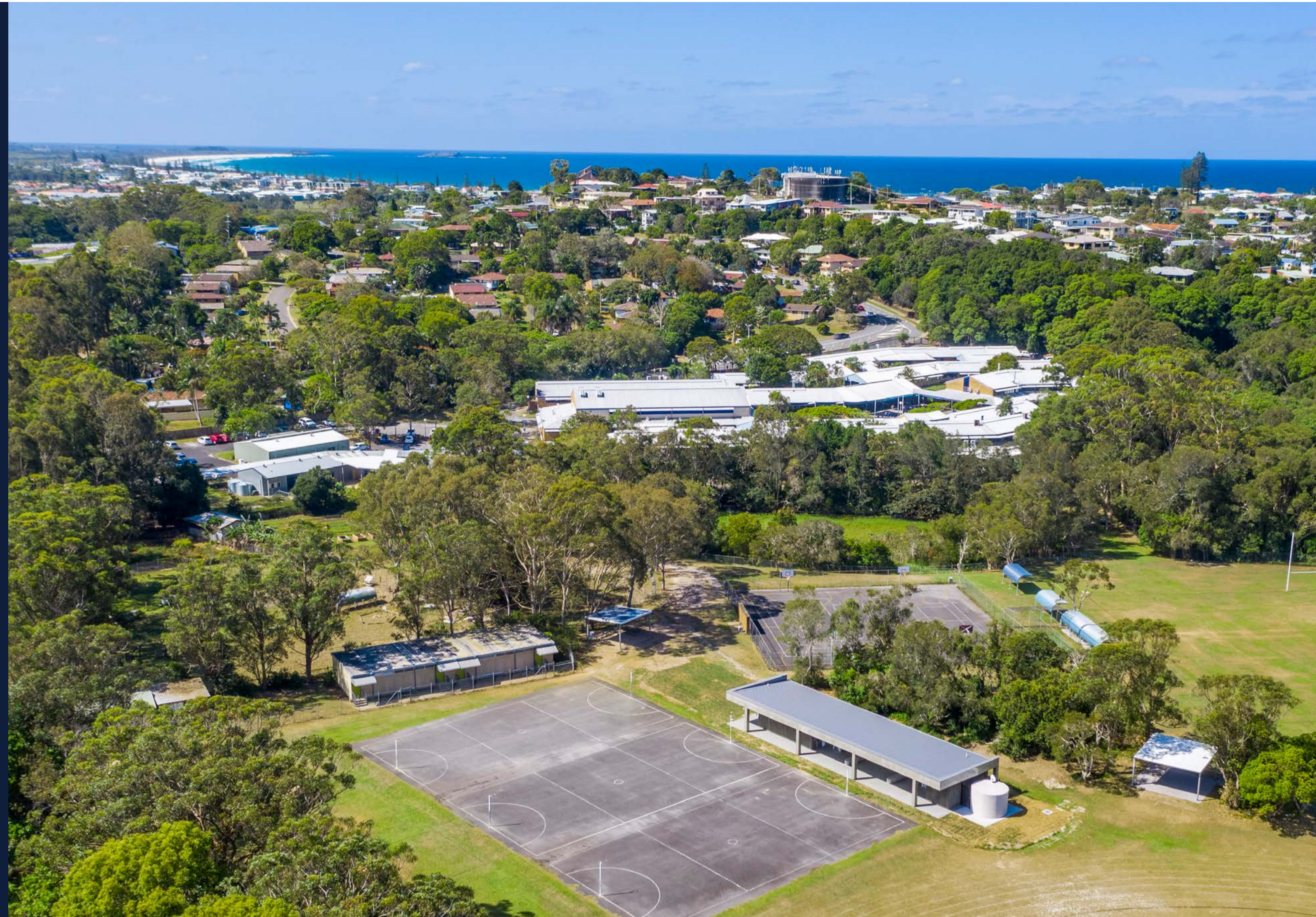
Aerial view of the Kingscliff High School upgrade
