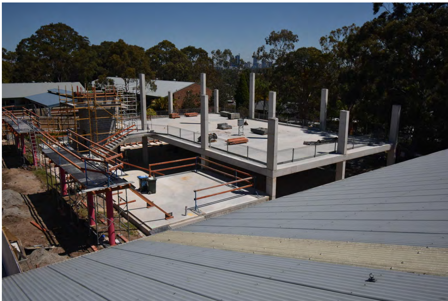
Killarney Heights Public School construction time lapse October 2019
