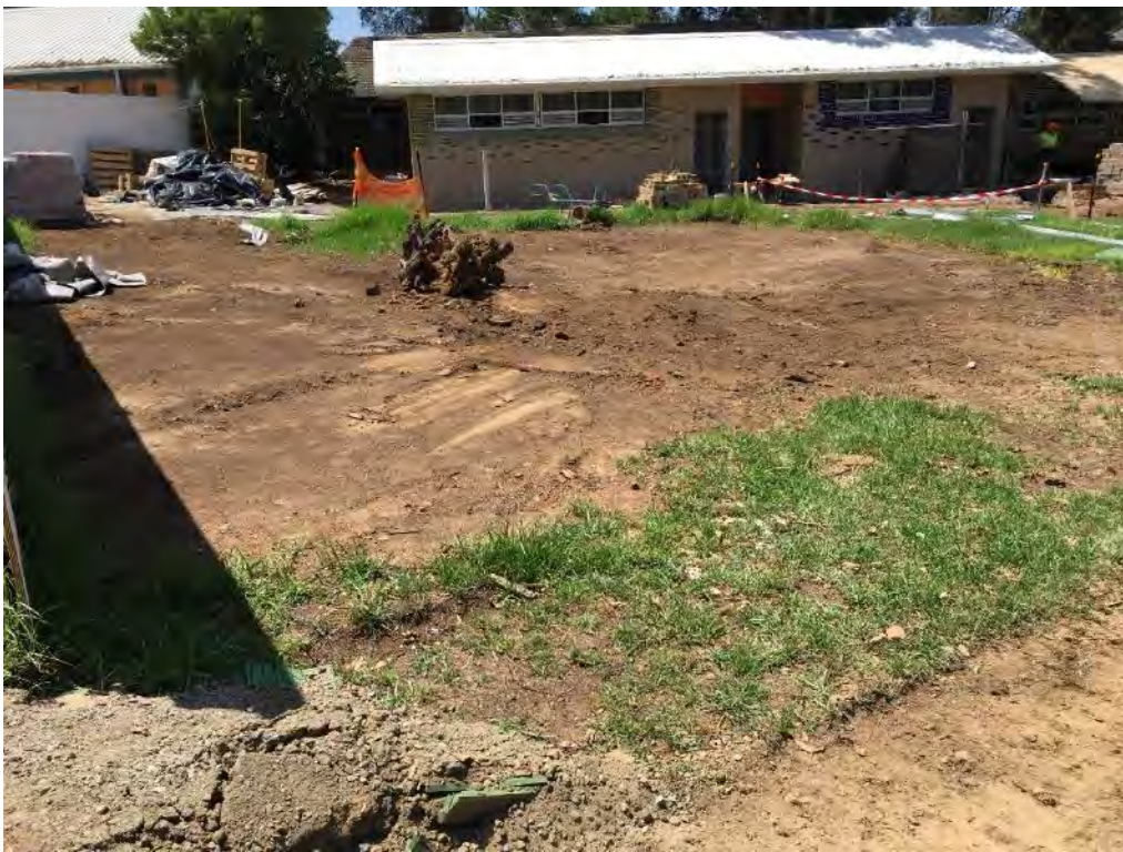
Photograph 3: Southern portion of clearance area - East facing (22/01/20)
