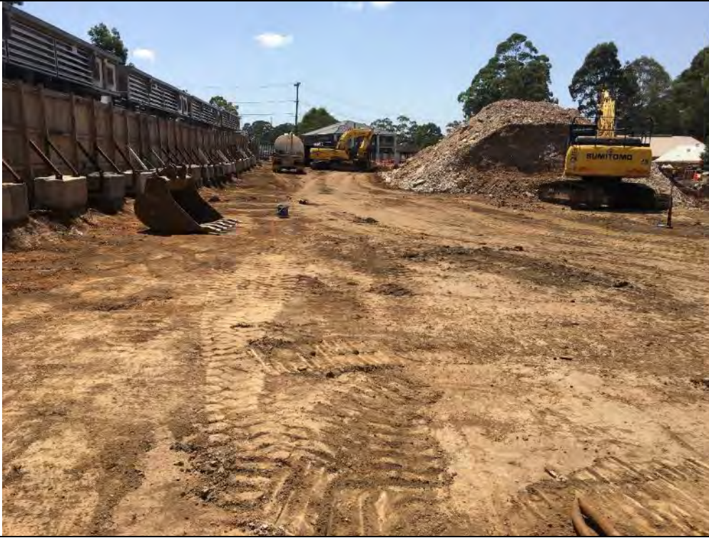
Photograph 5: Western portion of clearance area - North facing (22/01/20)
