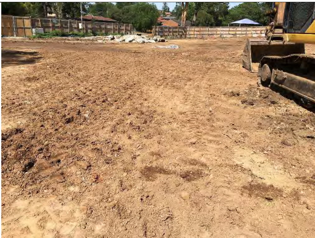
Photograph 9: Friable removal area - South facing (23/01/20)
