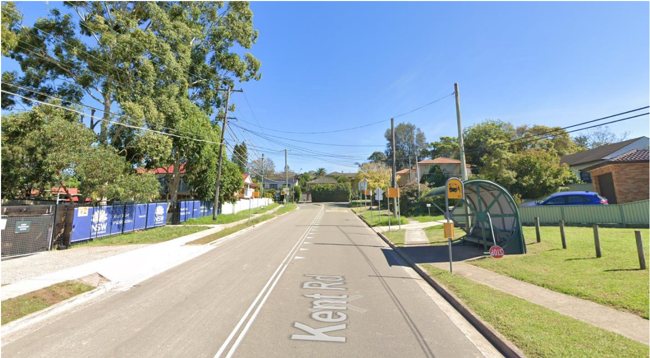
Figure 3.8: Bus stops at Kent Road
