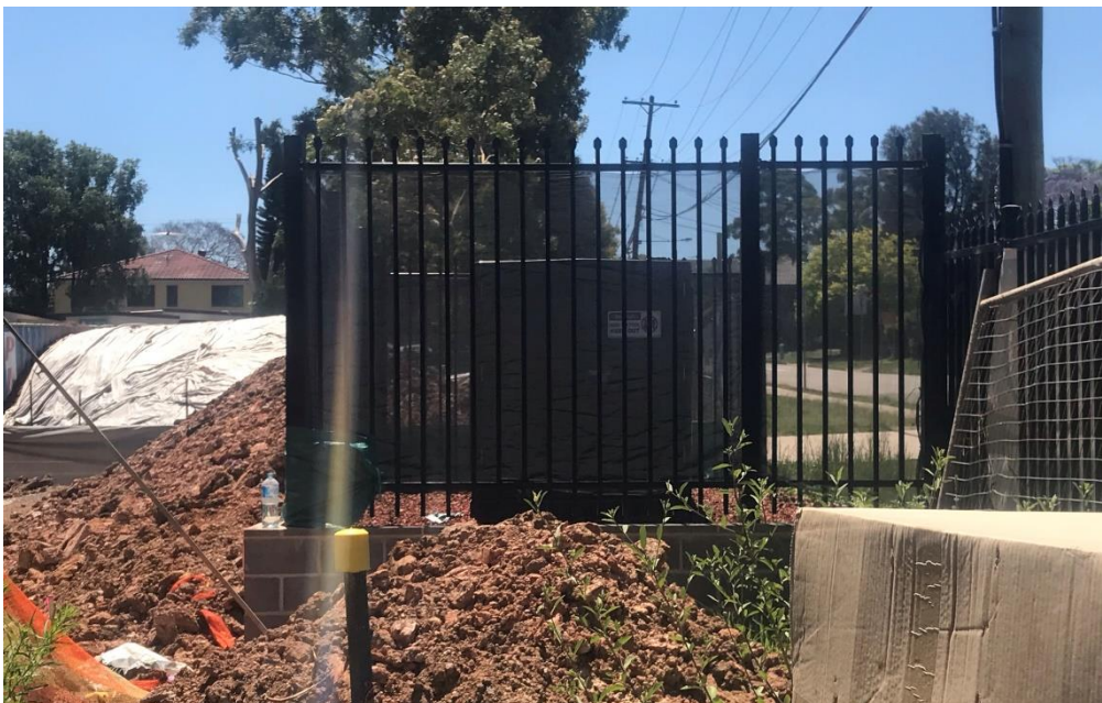
Figure 5: Stockpile at rear of site covered in geofabric and sediment fencing in place around perimeter of site
