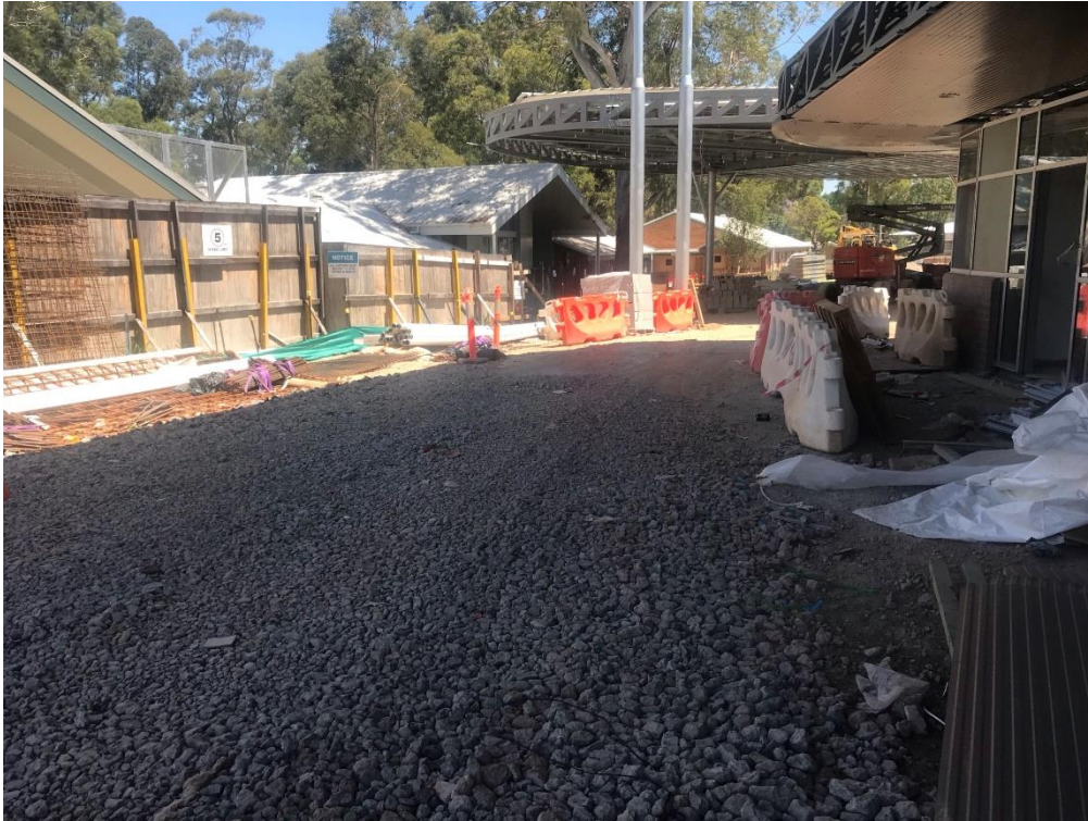
Figure 6: Gravel in place on site to prevent tracking of mud
