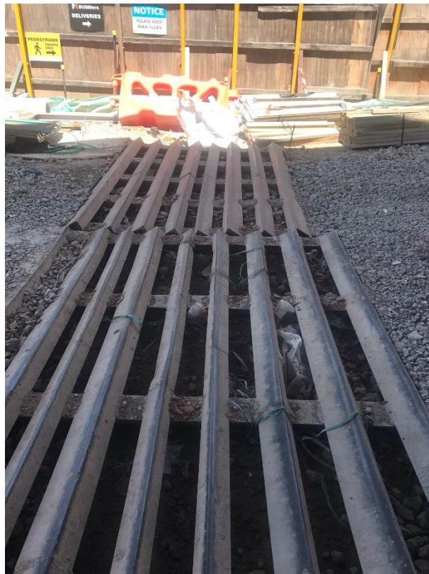
Figure 3: Cattle grid kept clean of debris
