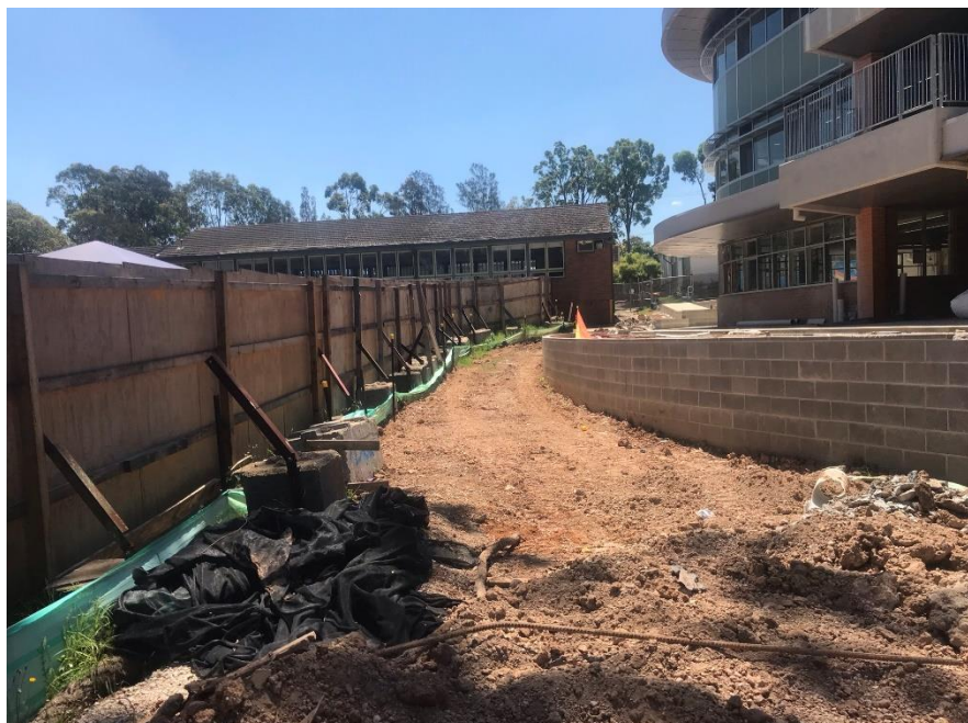
Figure 8: Sediment fence in place around entire site perimeter
