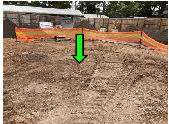
Photograph 4. Southern Stockpile Area – Following removal
