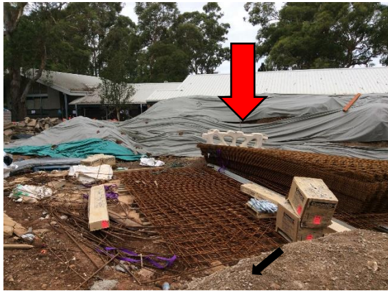
Photograph 1. Northern Stockpile – Prior to removal
