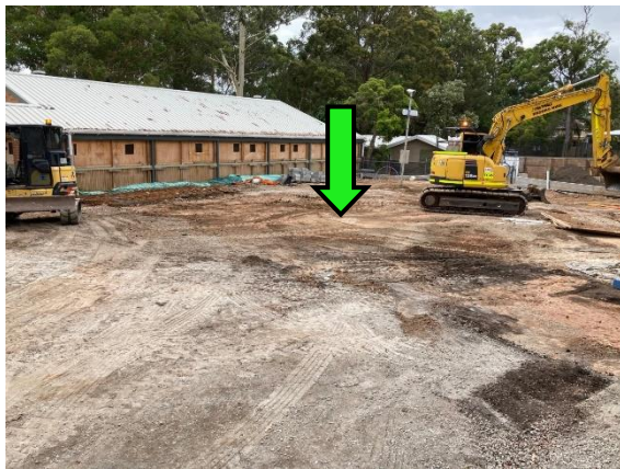
Photograph 3. Northern Stockpile Area – Following removal
