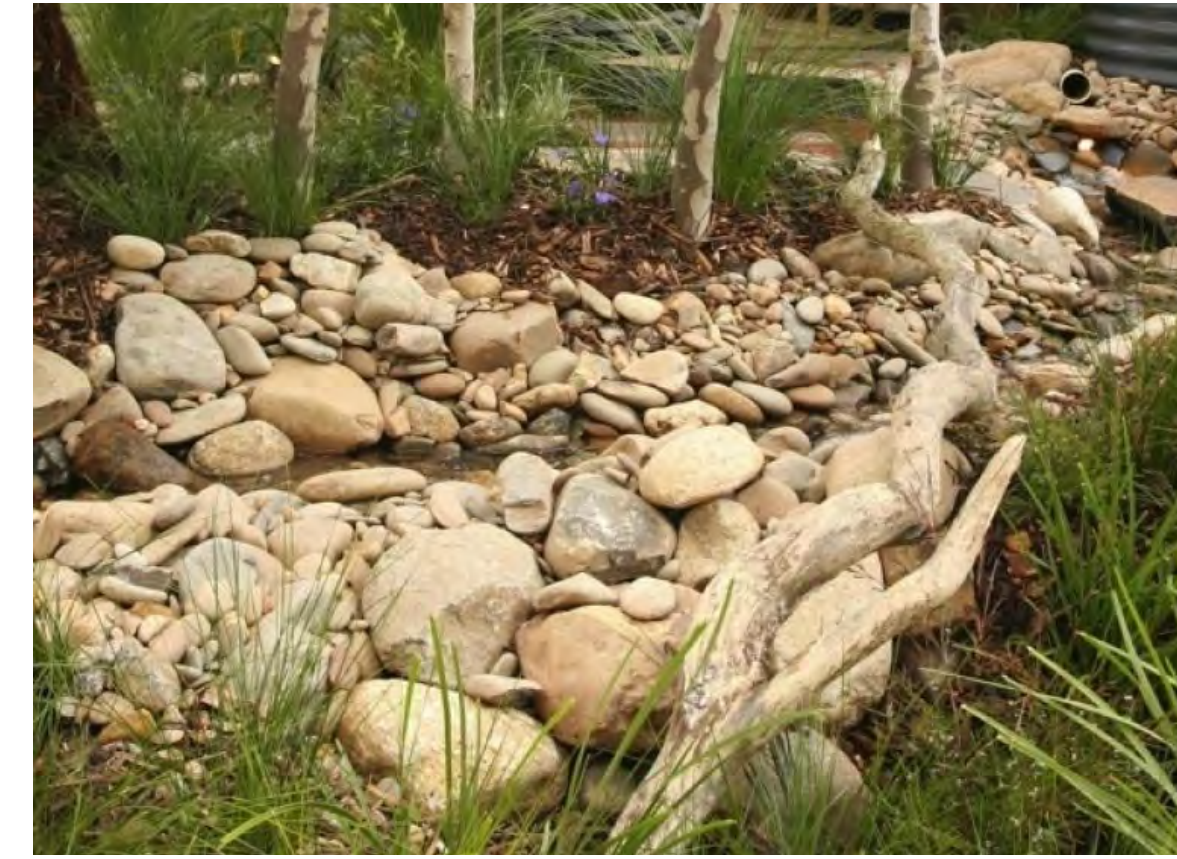
Planted sandstone spalls rain garden
