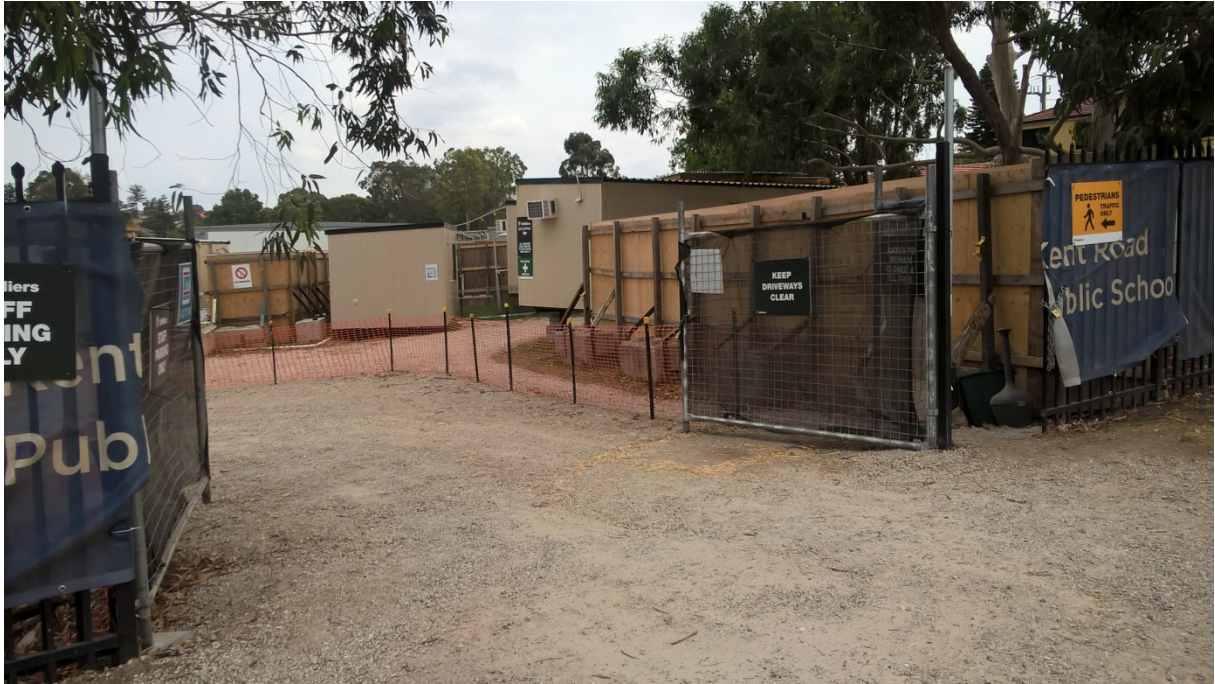
Figure 3: Pedestrian and truck access to site
