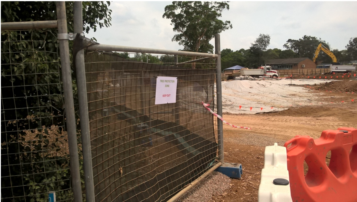
Figure 2: Tree protection measures in place
