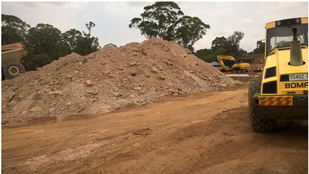
Figure 6: Excavated material stockpile located at the centre of the site
