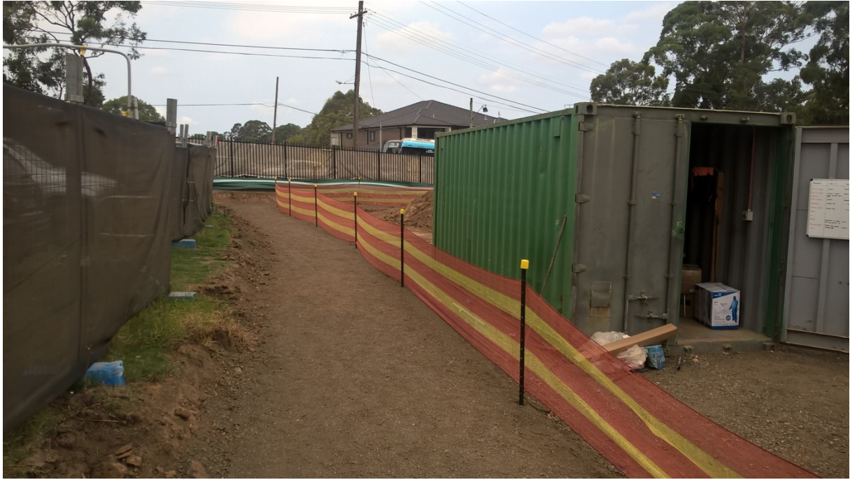
Figure 7 Internal hoarding and sediment fencing
