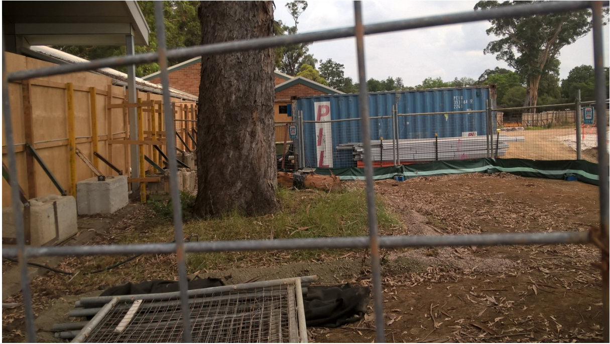
Figure 5: Tree protection zone in place to protect hollow for future use on-site
