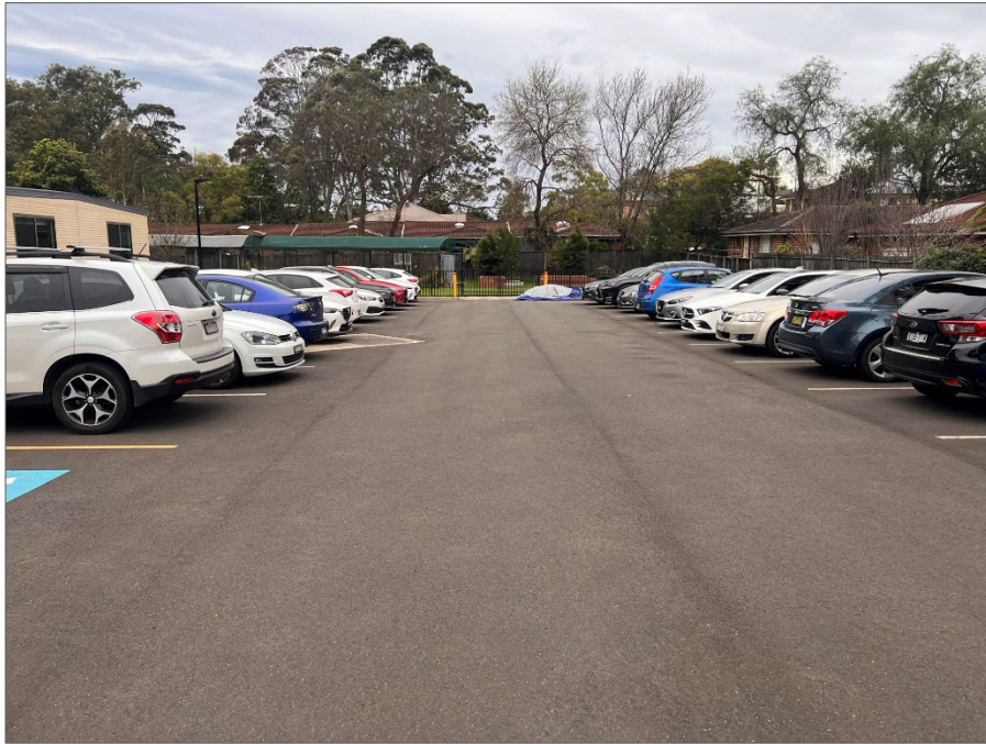
Figure 5: Extended carparking area constructed
