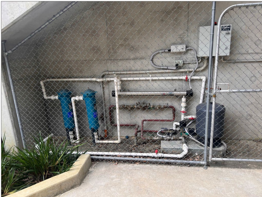
Figure 8: Water management facilities constructed
