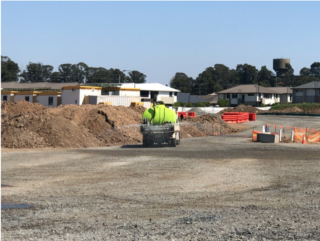
Figure 14 Water suppressant in use
