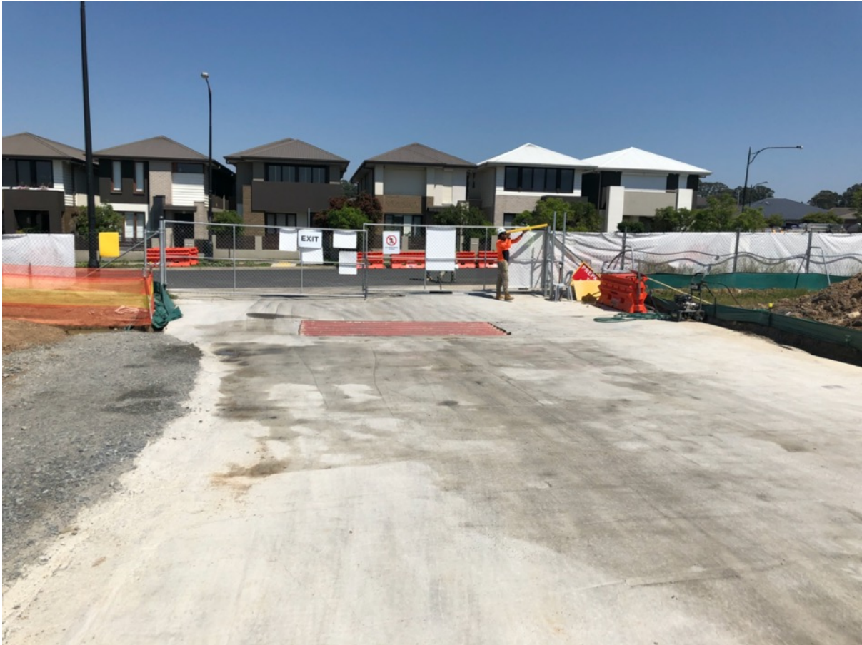
Figure 9 Entry/ exit point to site with rumble grid and wheel wash
