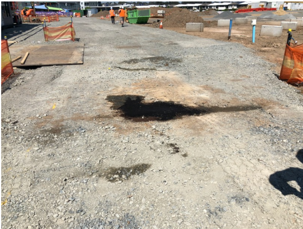
Figure 17 Hydraulic oil spill in process of being remediated
