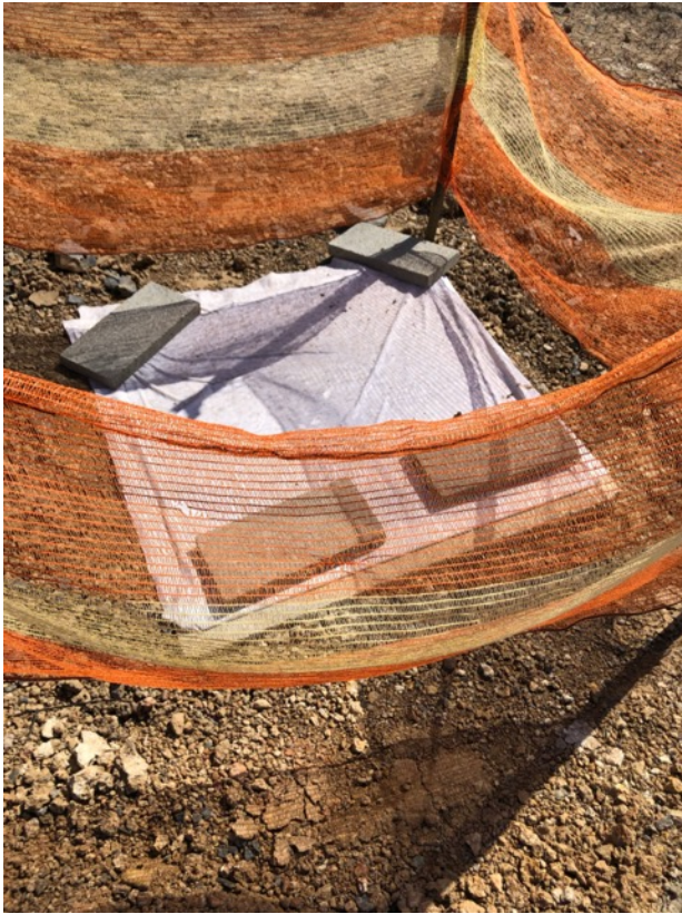
Figure 7 Sediment protection for stormwater grates
