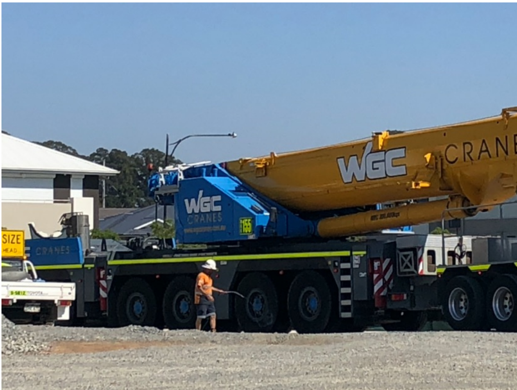
Figure 10 Wheel wash down prior to leaving site
