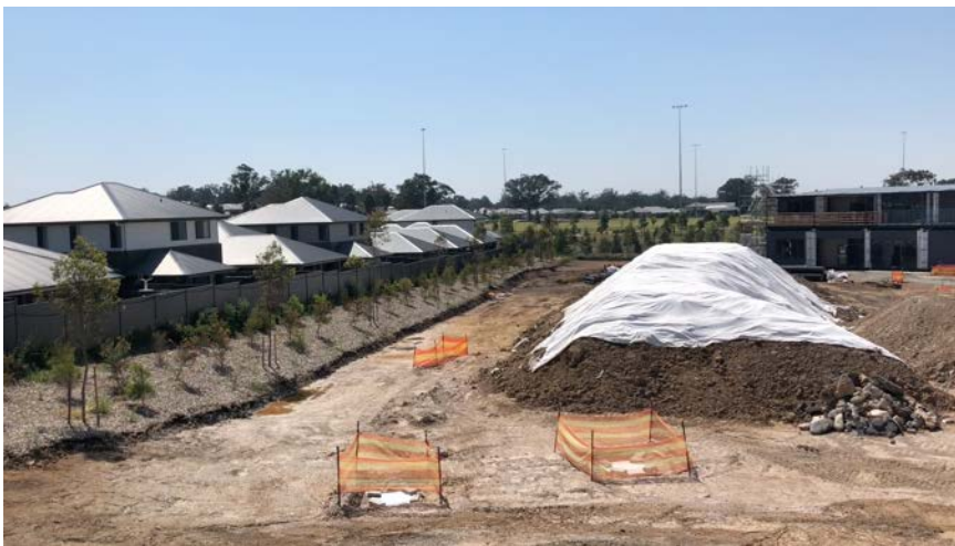
Figure 8 Stockpile stabilisation and erosion and sediment control
