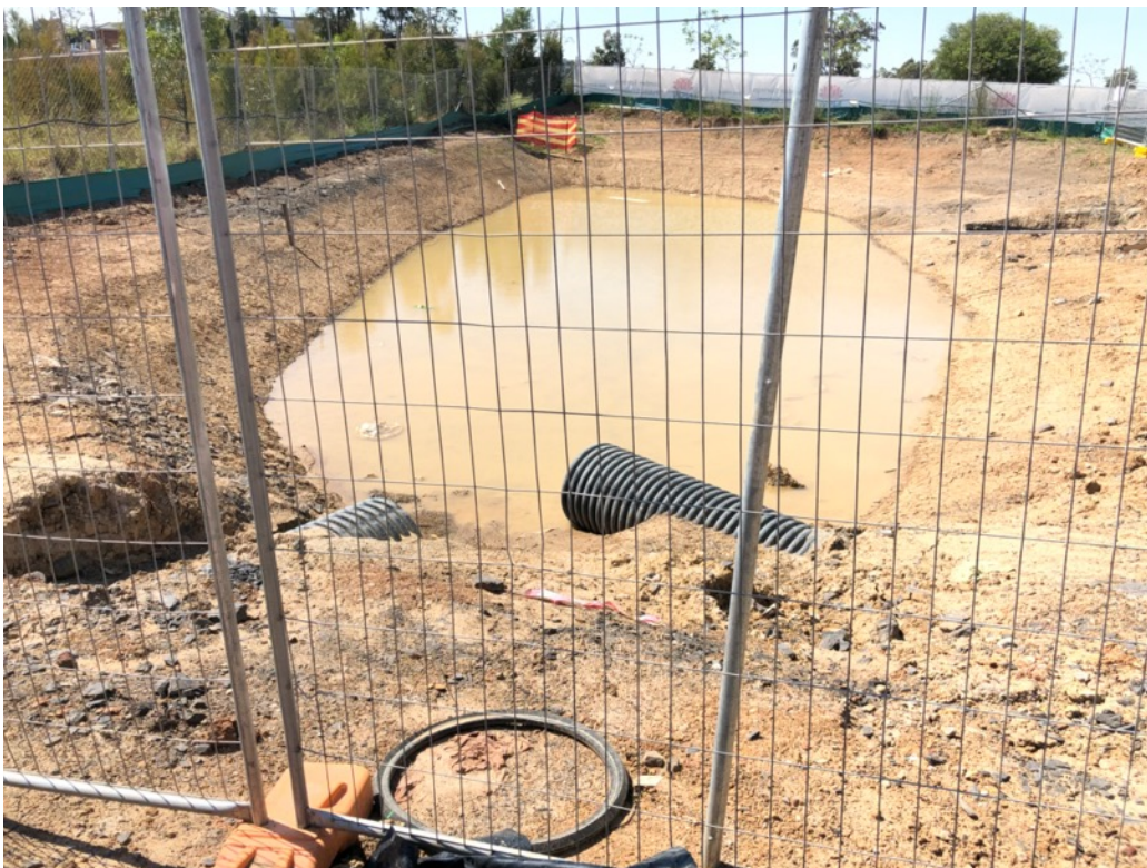
Figure 15 Sediment basin
