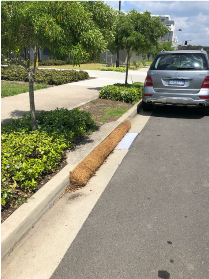
Figure 11 Sediment protection at entrance to site
