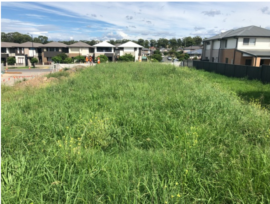
Figure 10 Vegetated and stabilised stockpile
