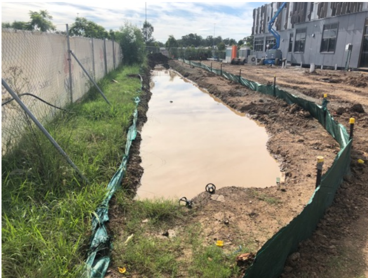
Figure 12 Effective erosion and sediment controls
