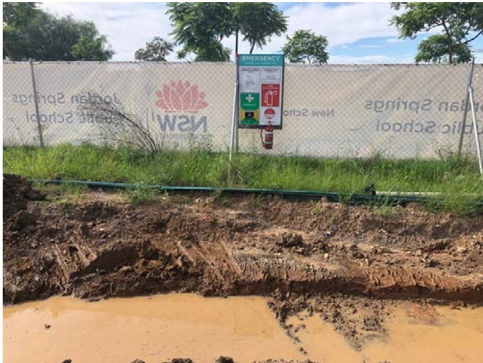
Figure 6 Low accessibility fire extinguisher
