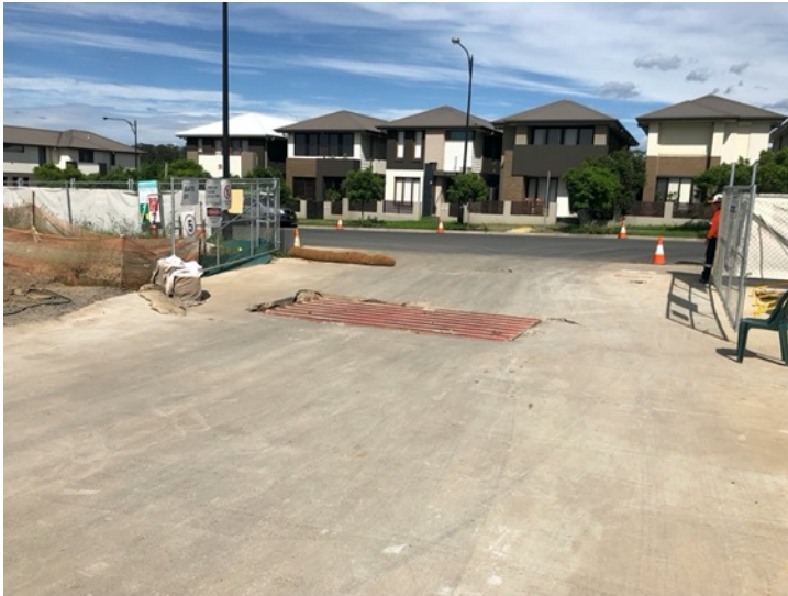
Figure 7 Entry/ exit point to site with rumble grid and wheel wash
