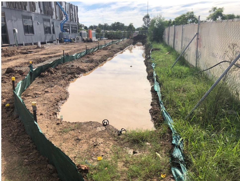
Figure 14 Boundary sediment controls - collapsed sediment curtain
