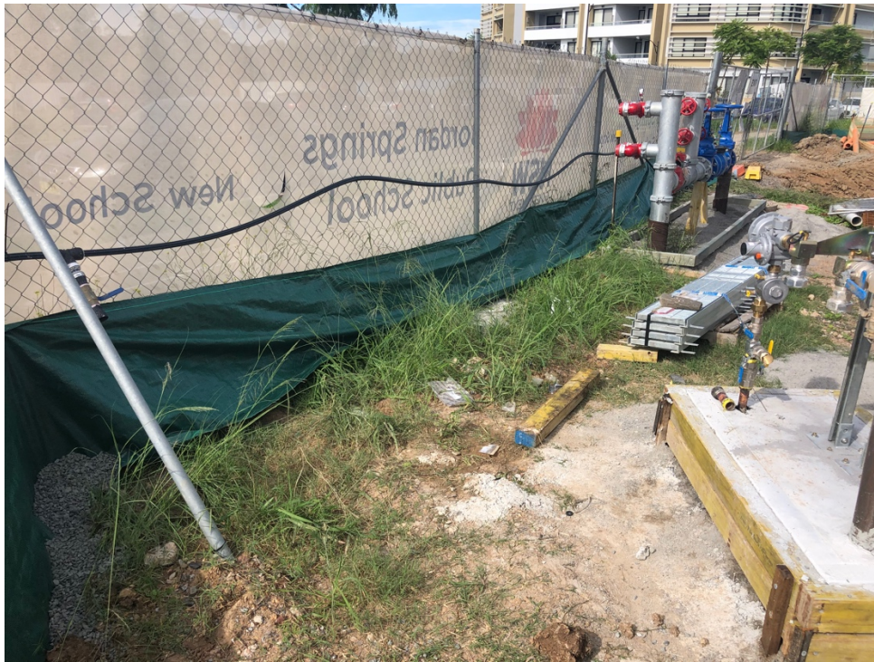
Figure 13 Boundary sediment controls - curtain above ground level
