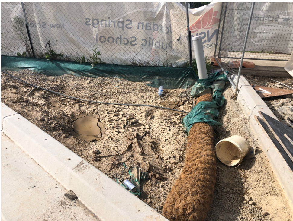
Figure 12 Boundary sediment controls
