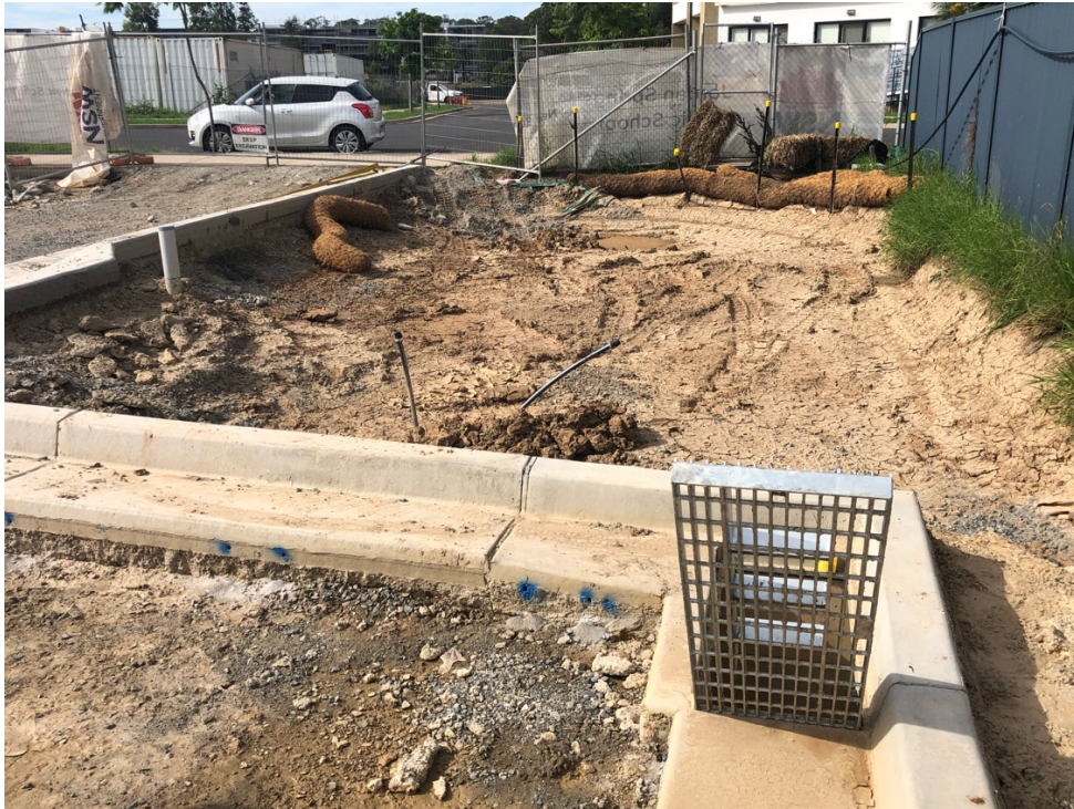
Figure 11 Boundary sediment controls - overtopped and displaced coir roll, saturated hay bales, collapsed sediment curtain.
