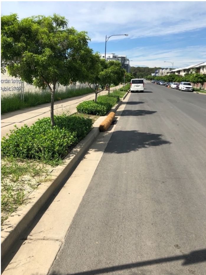
Figure 8 Sediment protection at entrance to site
