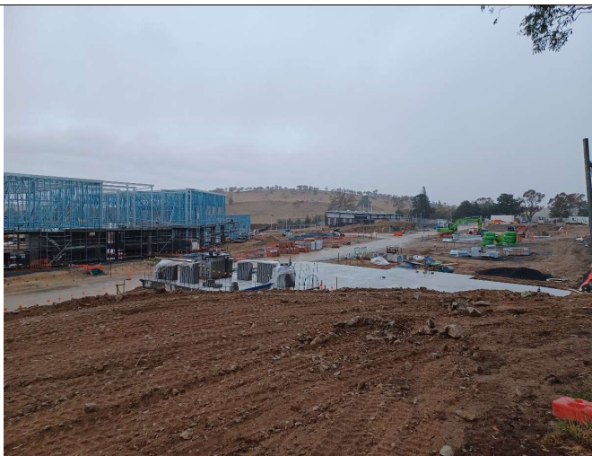
Photo 1: Looking south-east at the cleared Site.
