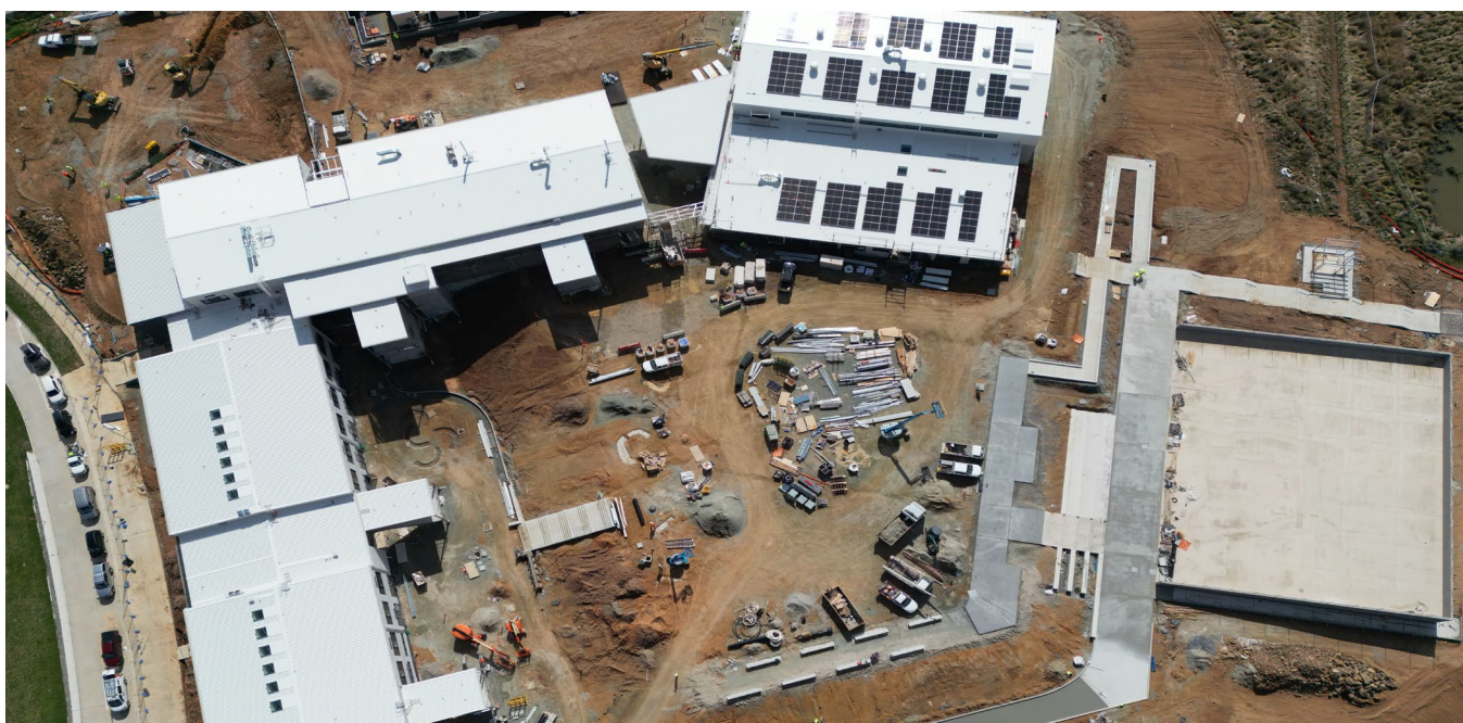
Drone photo of Jerrabomberra High School under construction
