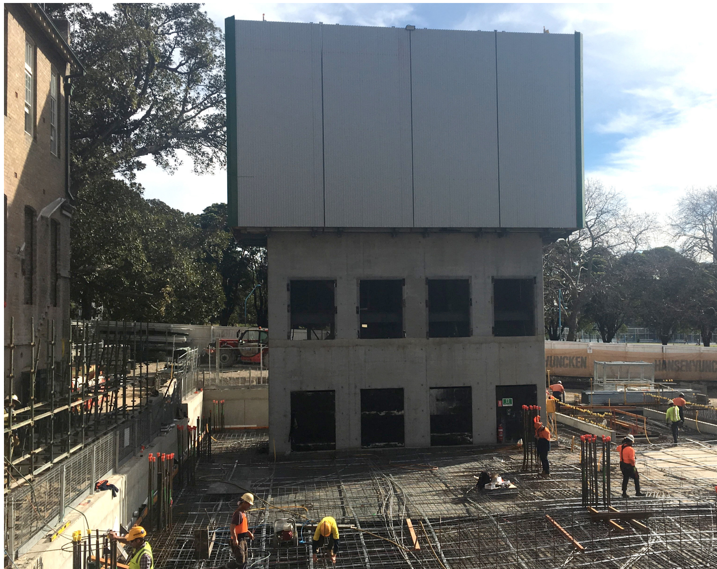
The new school's tower lift shaft is progressively rising from basement level
