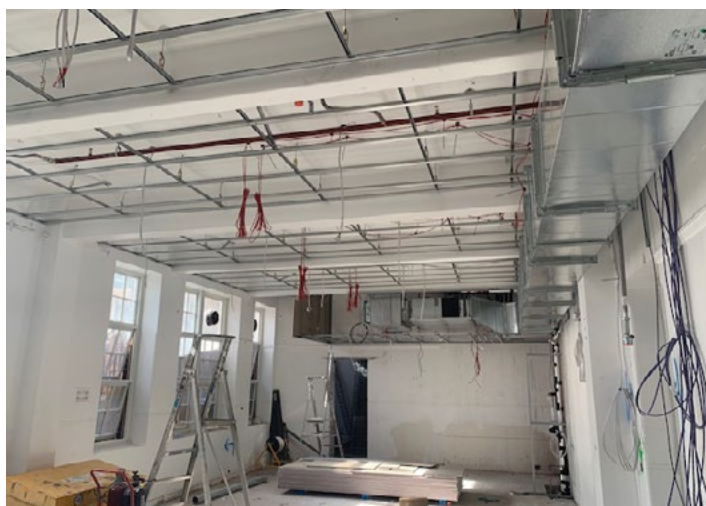
Extensive rewiring, specialist STEM fit-out, air-conditioning and installation of fire safety sprinklers is being incorporated in the existing heritage buildings
